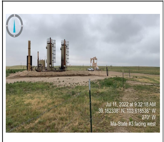
Photograph 4: West facing photograph.
