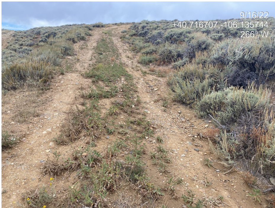
Photo 1. Photo shows the start of the Location access road. The road is not reclaimed; it is crowned, compacted and graveled. Vehicles appear to be utilizing it. The green vegetation in the center of the road is Canada thistle (CO List B Noxious).
