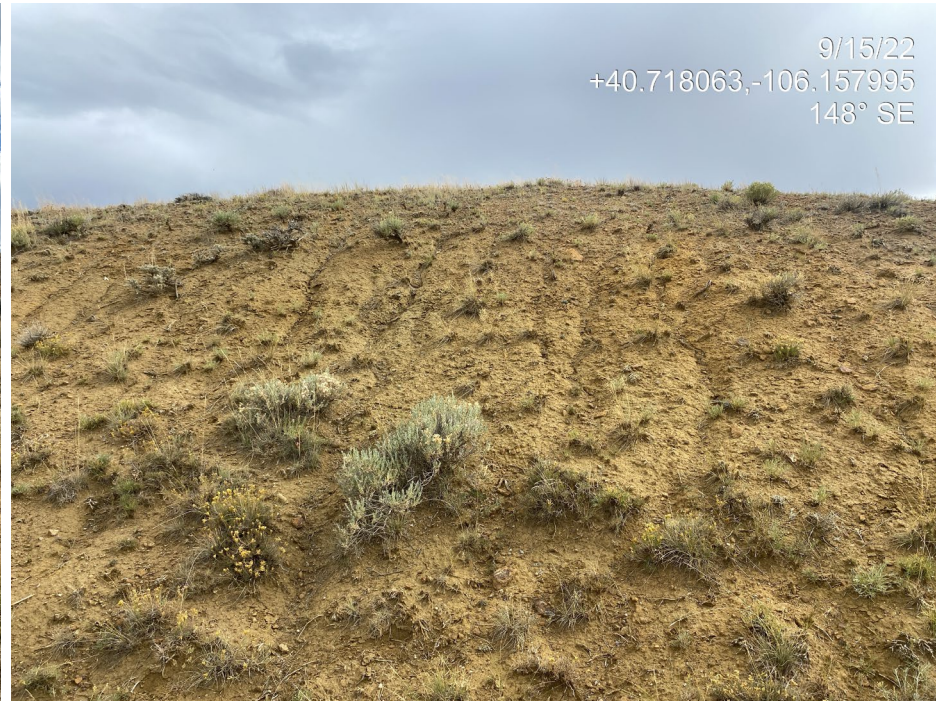
Photo 6. Photo shows rill erosion occurring on the cut slope at the south of the Location.
