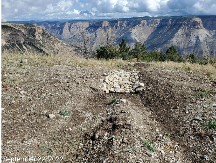
Photo 1: Photos taken from the sediment trap on the north end of the Location. Though work to maintain sediment trap has been conducted, work has not been conducted in accordance with good engineering practices; geotextile lining has not been installed at the inlets/outlets with the rip-rap material.
