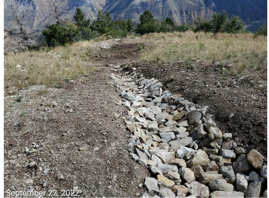
Photo 1: Photos taken from the sediment trap on the north end of the Location. Though work to maintain sediment trap has been conducted, work has not been conducted in accordance with good engineering practices; geotextile lining has not been installed at the inlets/outlets with the rip-rap material.
