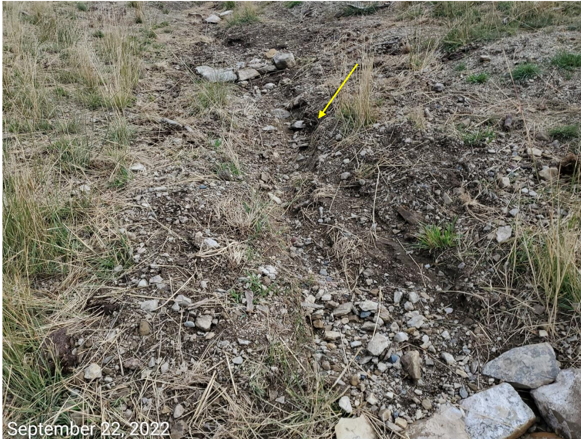
Photo 7: Photo example showing recurring stormwater erosion within the ditch.
