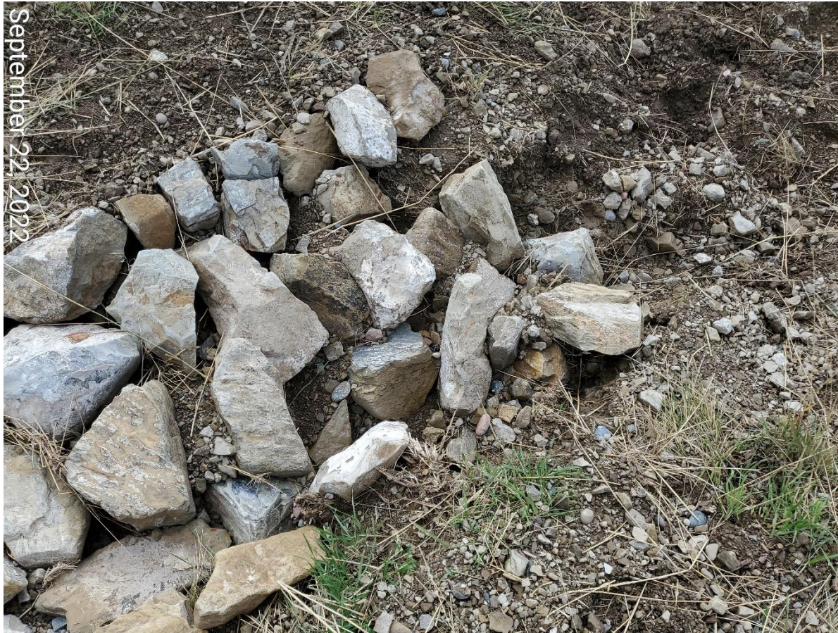
Photo 2: Continue from photo 1. Photo shows Operator installed rock (rip-rap) to armor inlet, however, geotextile lining has not been used as part of the armoring in accordance with good engineering practices, resulting in recurring stormwater degradation beneath and around the rip-rap material.
