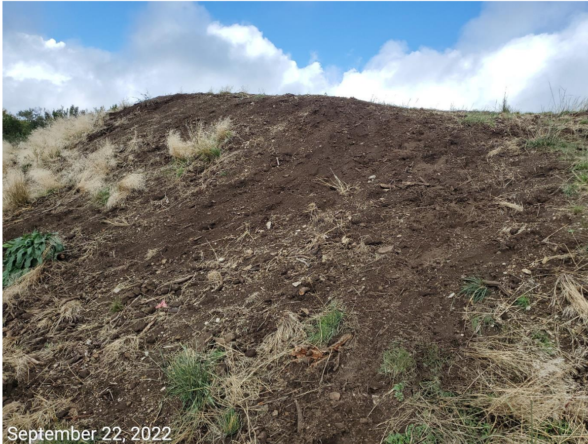
Photo 9: Photo taken from the southern slope of the southwester sediment trap. Photo shows work to repair the erosion degradation has been conducted, however soils have been left exposed and at risk to erosion; BMPs to stabilize soils until long term stabilization is achieved have not been installed.
