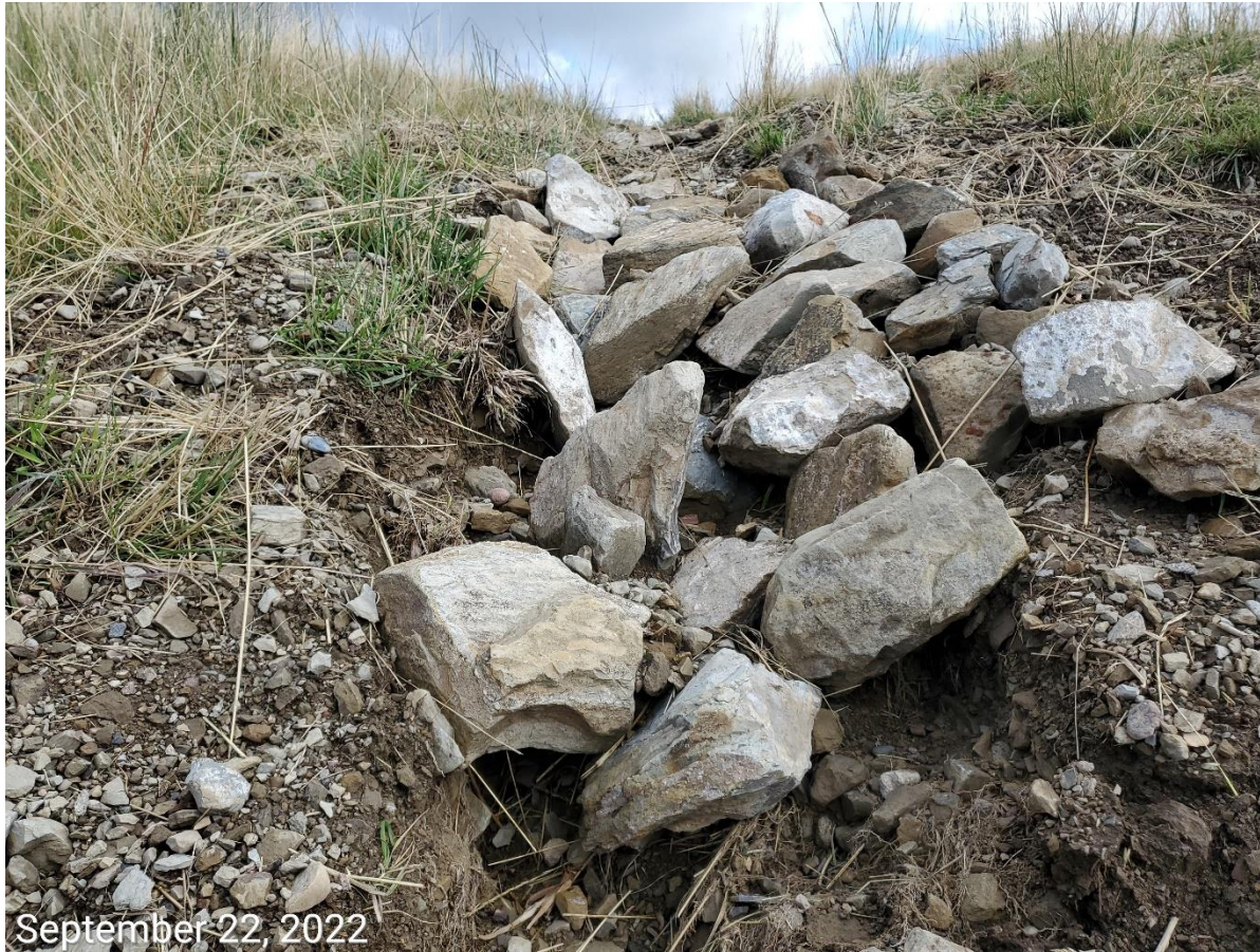
Photo 3: Continue from photo 2. Photo shows Operator installed rock (rip-rap) to armor inlet, however, geotextile lining has not been used as part of the armoring in accordance with good engineering practices, resulting in recurring stormwater degradation beneath and around the rip-rap material.
