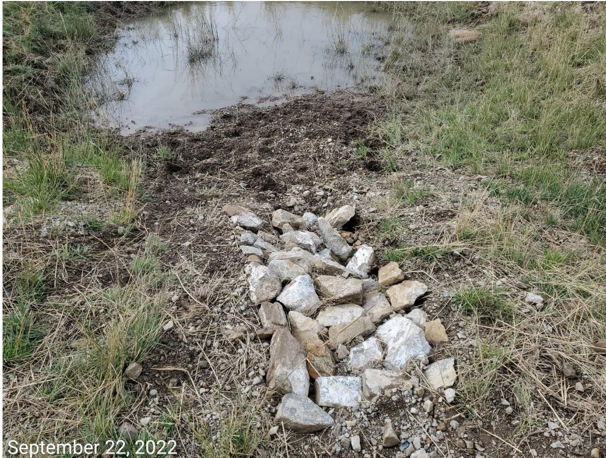
Photo 1: Photo taken from the sediment trap on the southwest end of the Location. Photo shows Operator repaired the gully erosion and installed rock (rip-rap) to armor the inlet.
