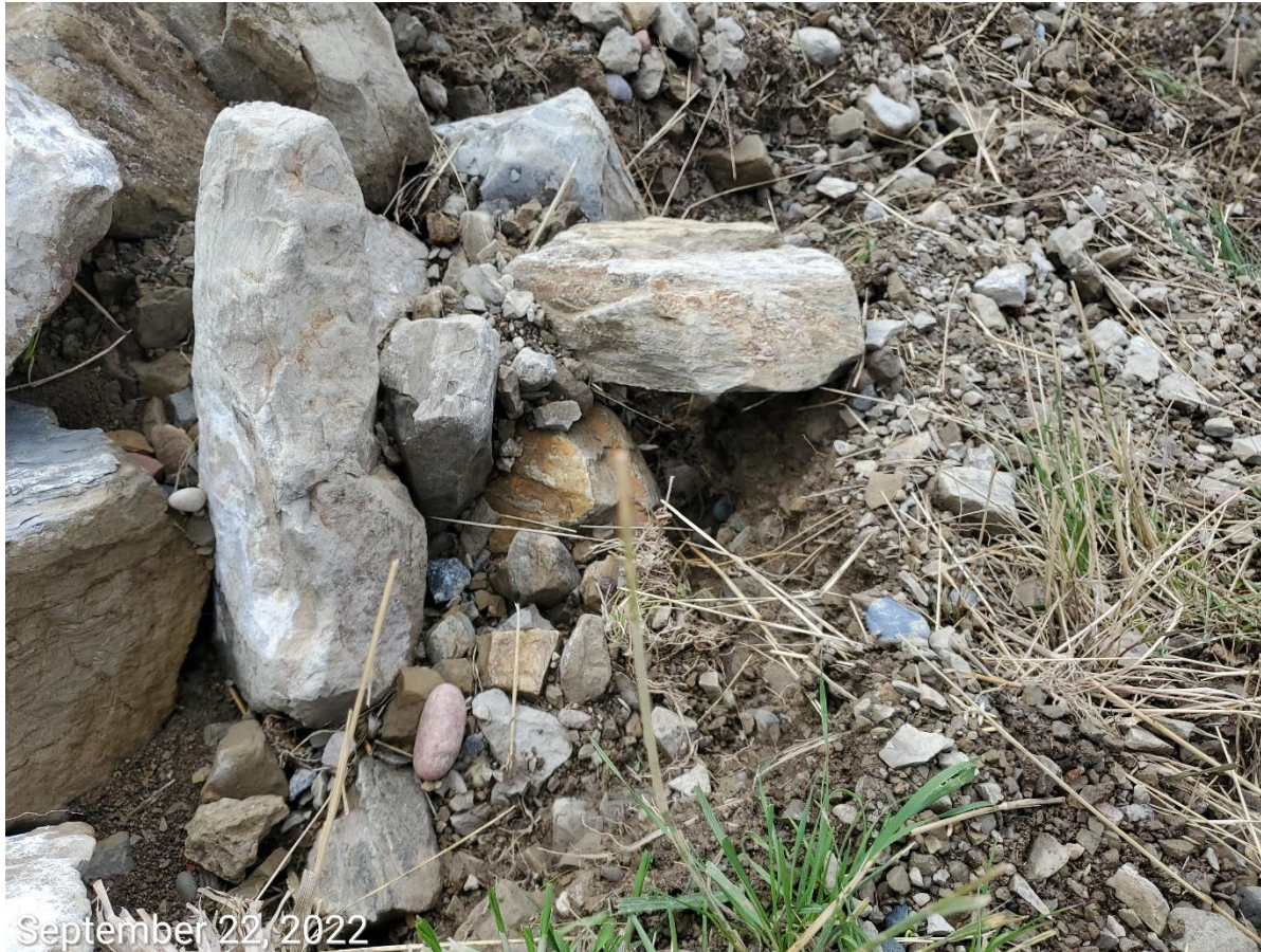
Photo 4: Continue from photo 3. Photo shows Operator installed rock (rip-rap) to armor inlet, however, geotextile lining has not been used as part of the armoring in accordance with good engineering practices, resulting in recurring stormwater degradation beneath and around the rip-rap material.
