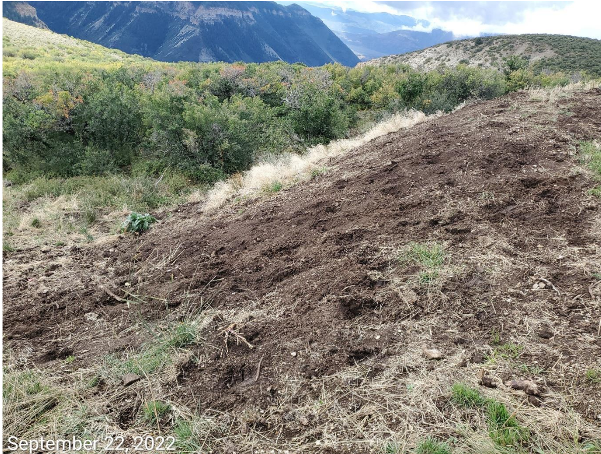
Photo 8: Photo taken from the southern slope of the southwester sediment trap. Photo shows work to repair the erosion degradation has been conducted, however soils have been left exposed and at risk to erosion; BMPs to stabilize soils until long term stabilization is achieved have not been installed.
