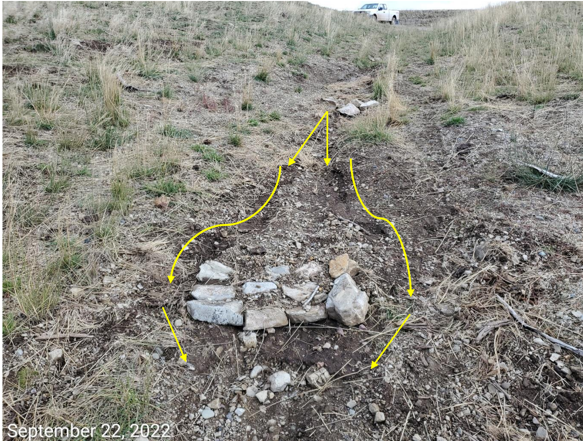
Photo 5: Photo shows rock-checks installed along ditch leading from the southwest end of the Location, leading to the sediment trap observed in photo 1. Rock-checks appear to be inadequate and not per good engineering. Arrows show stormwater appears to be traveling around the checks resulting in further degradation.
