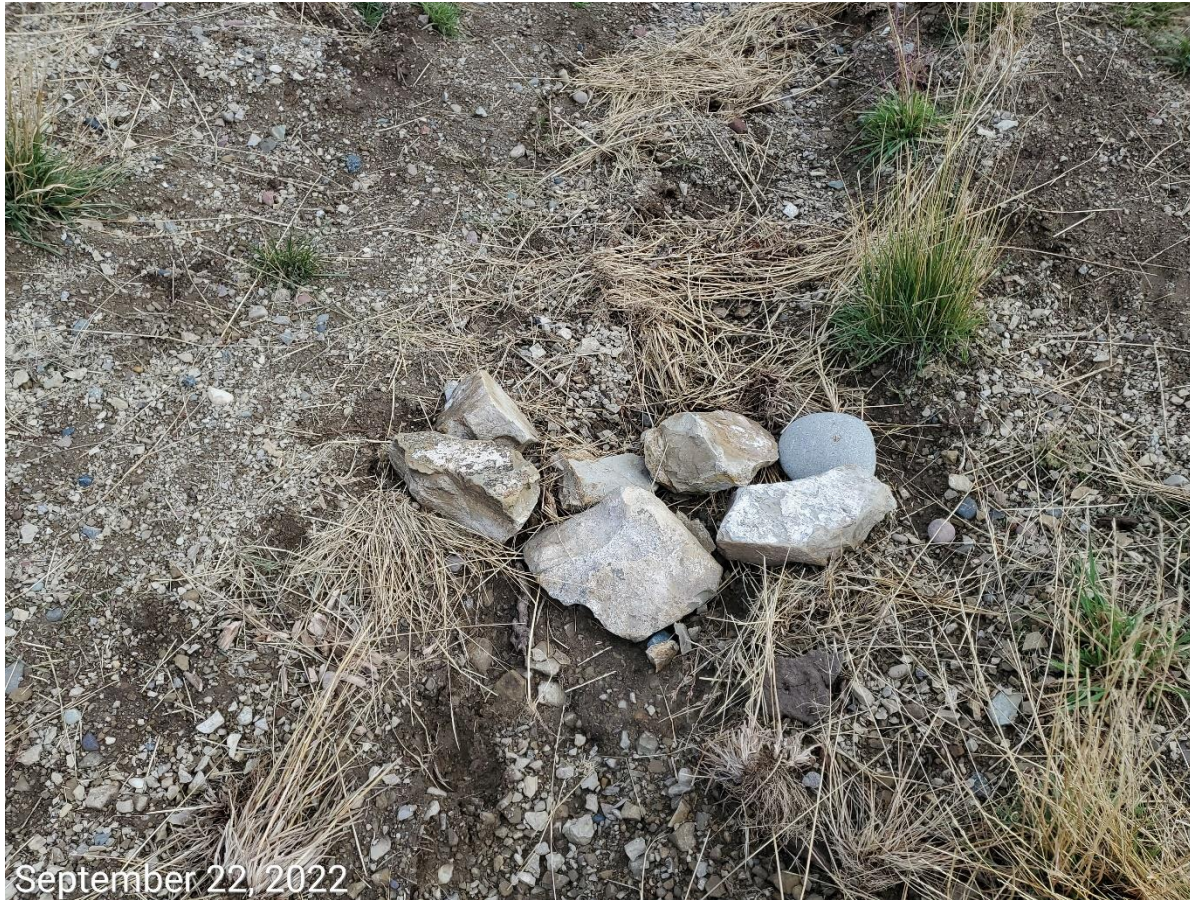
Photo 6: Photo shows example of rock-checks within ditch. BMP is not per good engineering practices and will facilitate degradation within the diversion ditch.
