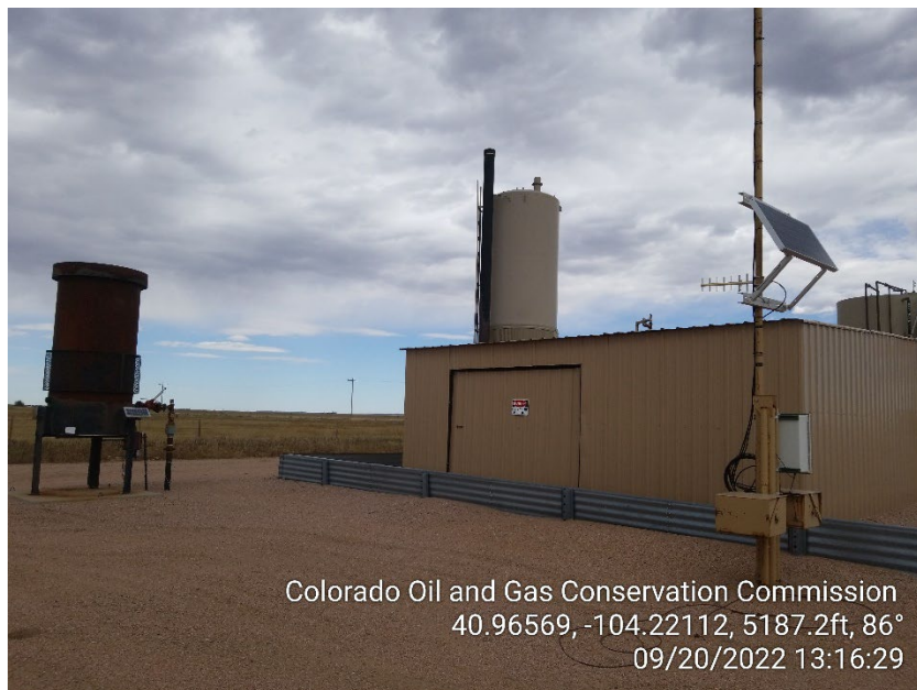
Photo 1 – Heater Treater and ECD
