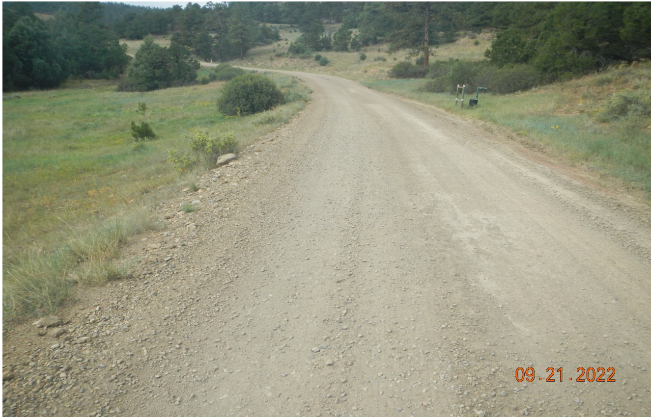
Photo 1. Facing south along the main access road.
