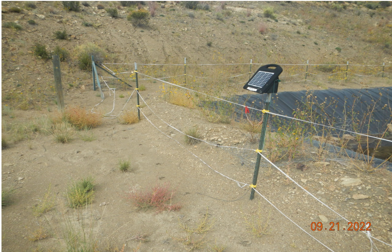
Photo 2. The fence around the pit is not maintained. May need to consider more robust fencing around lined pits.
