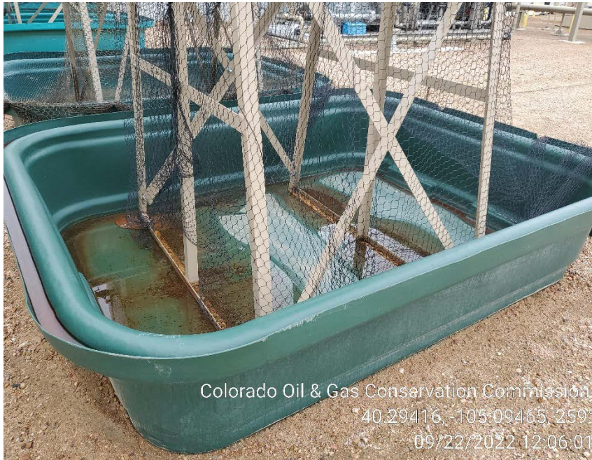
Bulk lube oil storage wildlife netting
