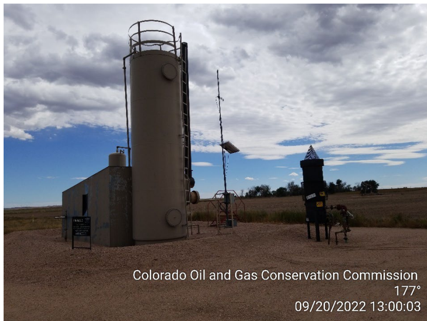
Photo 1 – Heater Treater and ECD
