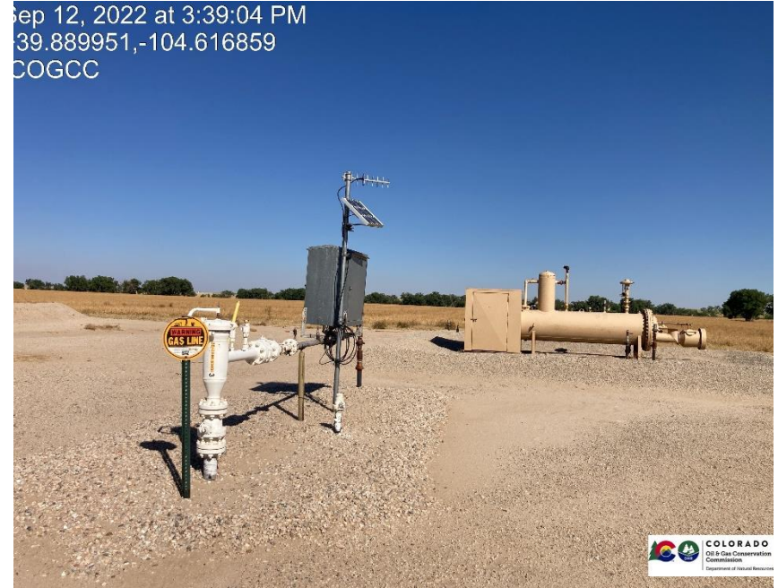
Pic 2 Separator gas meter run
