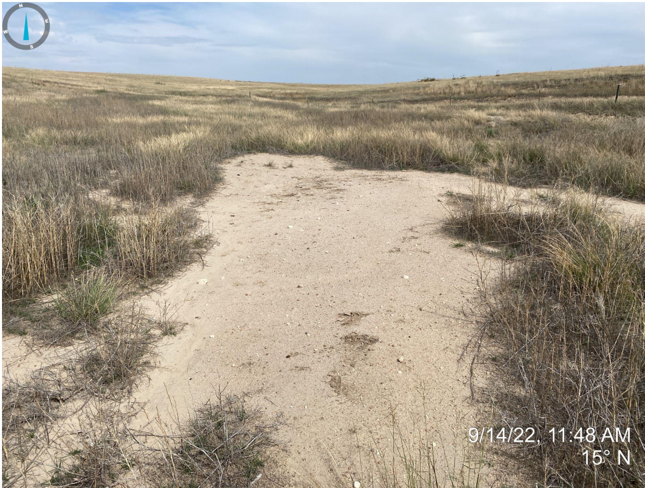
Photo 4. Taken from center portion of location, facing north. Photo illustrates location has not been reclaimed with lack of uniform vegetation cover (e.g. bare soil) and areas that have not been contoured and regraded to reflect reference areas.
