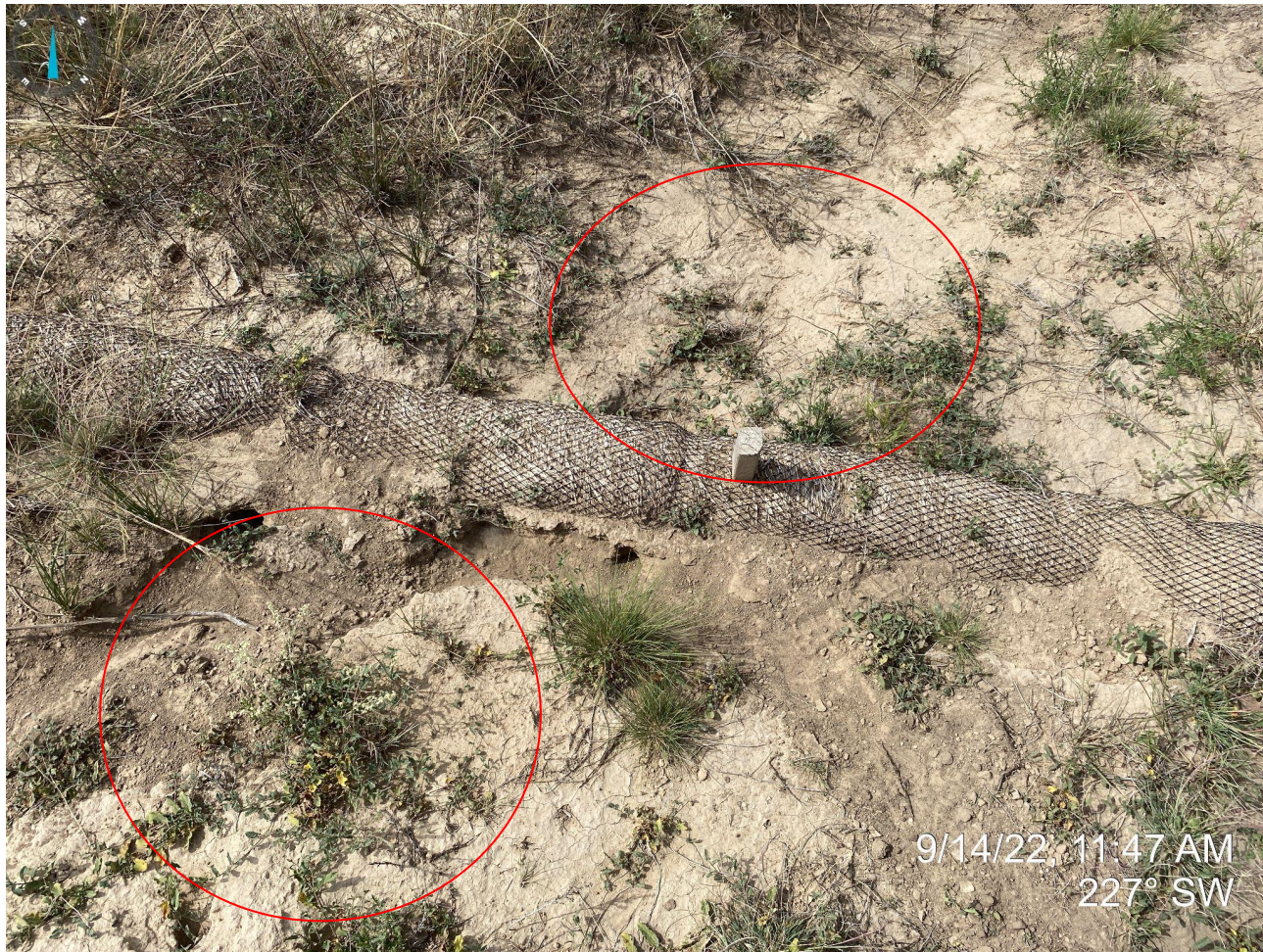
Photo 3. Close up photo of straw wattle, which is now considered debris and needs to be removed, and field bindweed (CO List C Noxious Weed) outlined in red.
