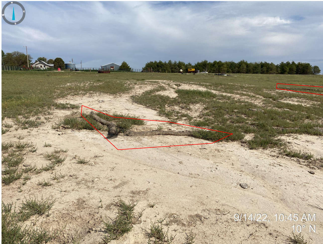
Photo 6. Facing north; degraded and/or improperly installed straw wattles outlined in red. These are considered debris and need to be disposed of properly.
