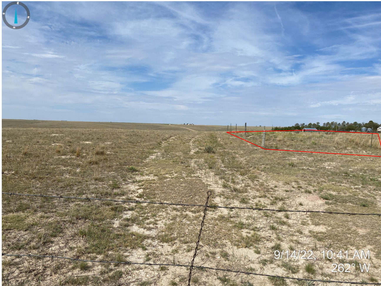
Photo 1. Taken from county road, facing west. Photo illustrates that access road has not been reclaimed and perimeter fencing is still installed (outlined in red); this is considered debris and needs to be disposed of properly.
