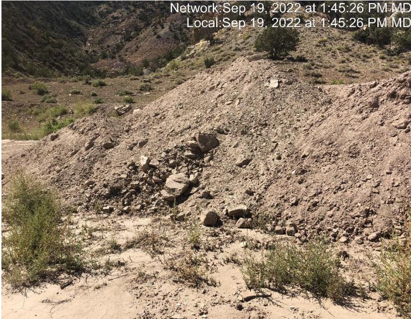
Photo #7735 BMP's have not been implemented around stockpiled soils.
