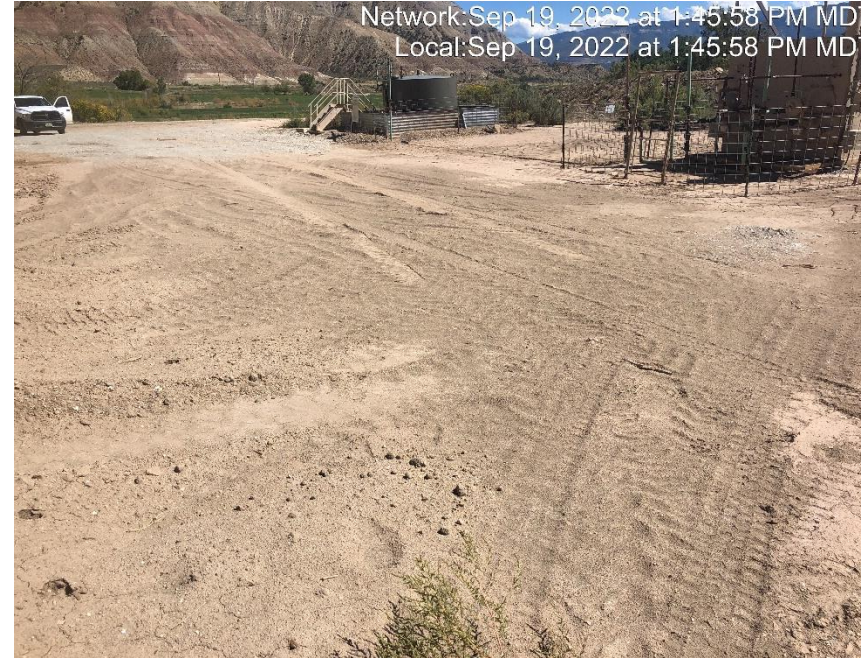
Photo #7739 BMP's have not been implemented around stockpiled soils.
