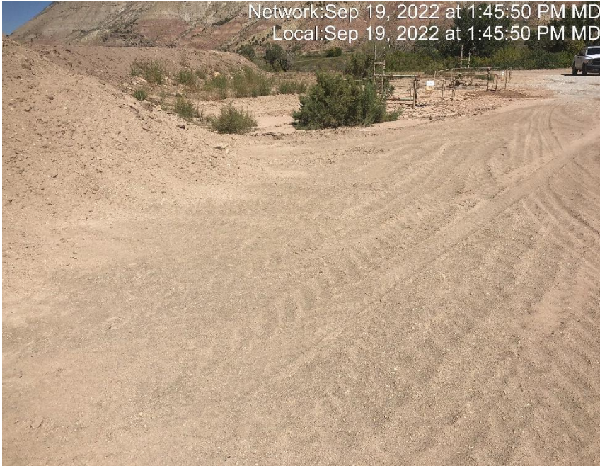
Photo #7738 BMP's have not been implemented around stockpiled soils.
