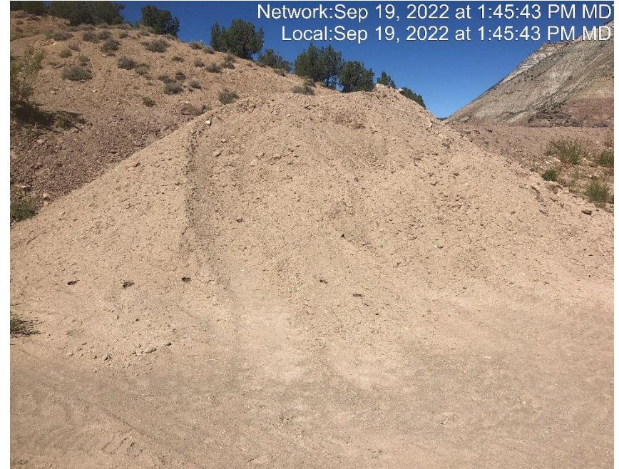
Photo #7736 Soils covering BMPs have not been implemented.
