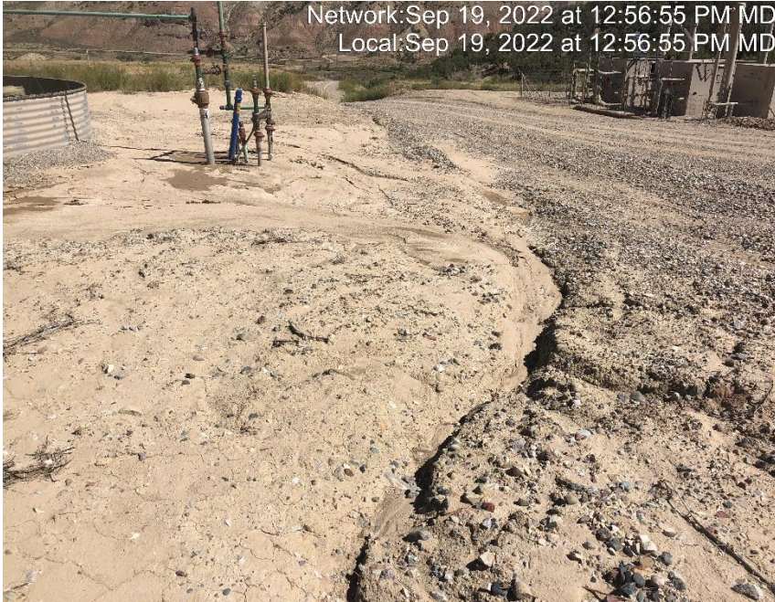
Photo #7715 Run on to location is not being controlled.
