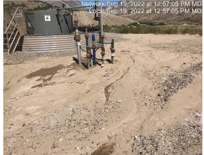
Photo #7716 Sediment is encroaching on equipment.
