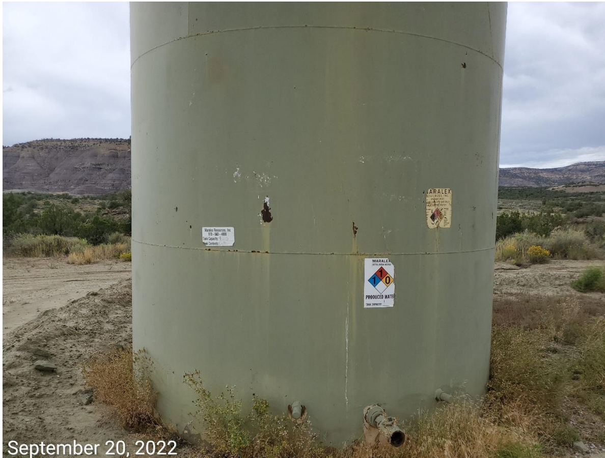
Photo 6: Labeling on tank does not comport with Rule 605.h
