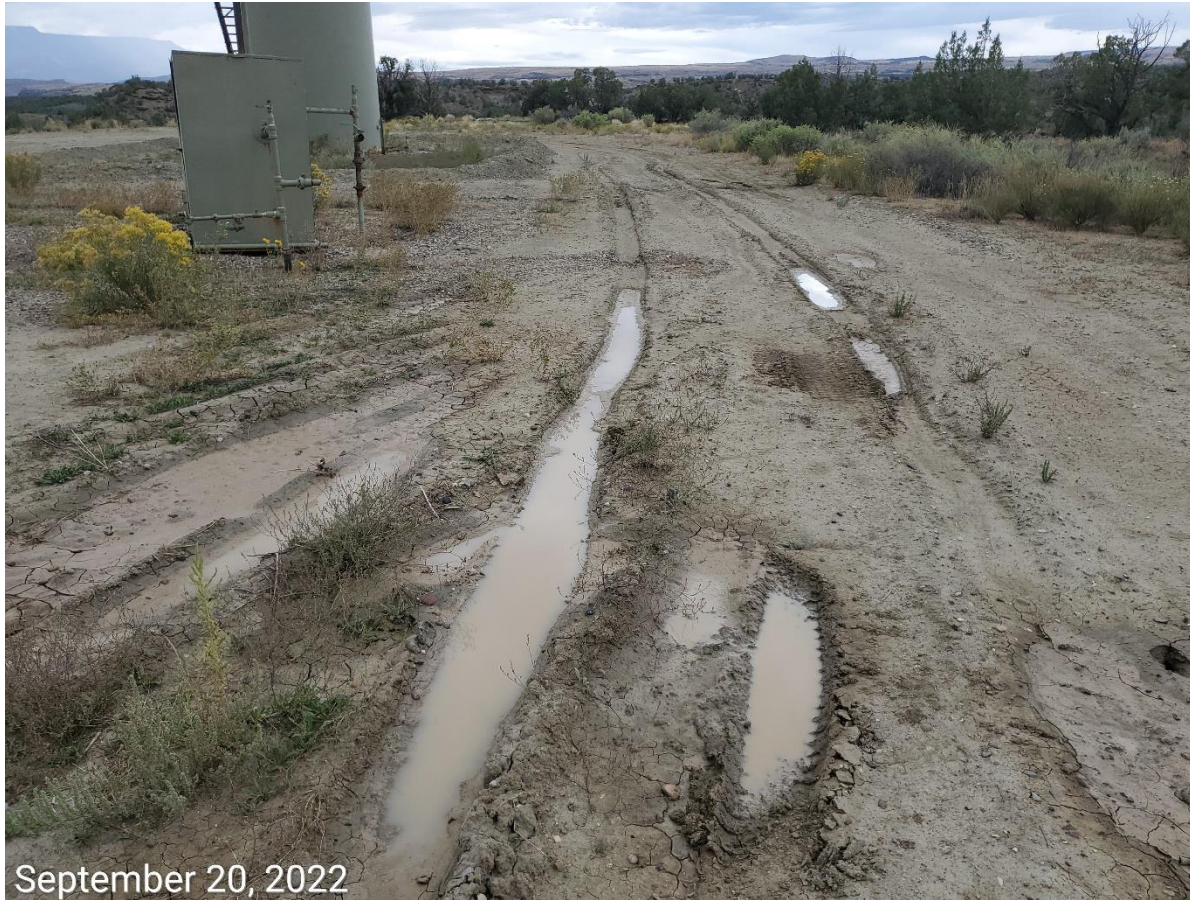
Photo 3: Photo example showing BMPs to stabilize the Location, and to minimize tracking and sediment transport remain missing or insufficient.
