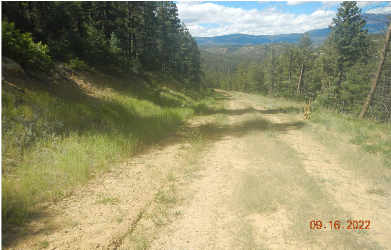
Photo 1. Facing northwest along the access road. The road had been regraded to repair erosion.
