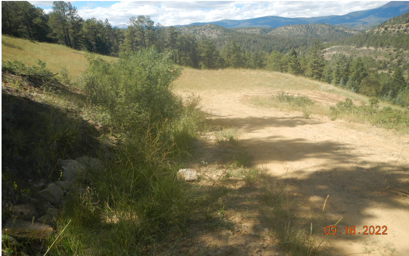
Photo 2. Facing northwest along the access road. The road had been regraded to repair erosion. Ongoing maintenance will be needed.
