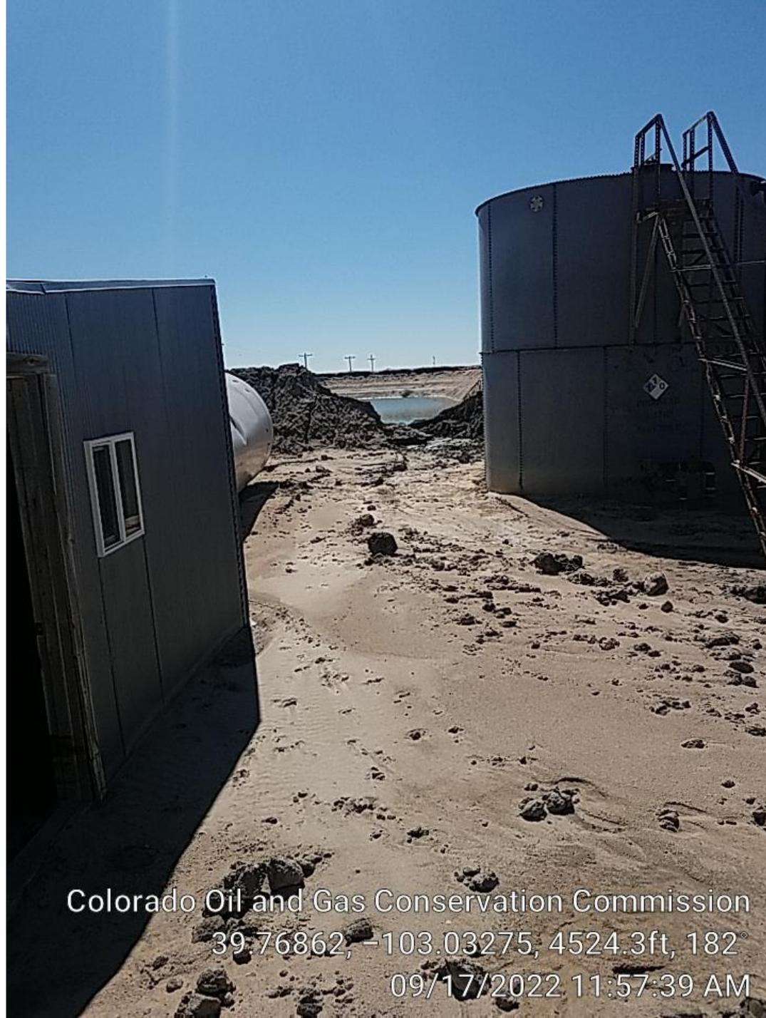
Same breach wall on east pit ran into treater shed and over secondary containment to the north.
