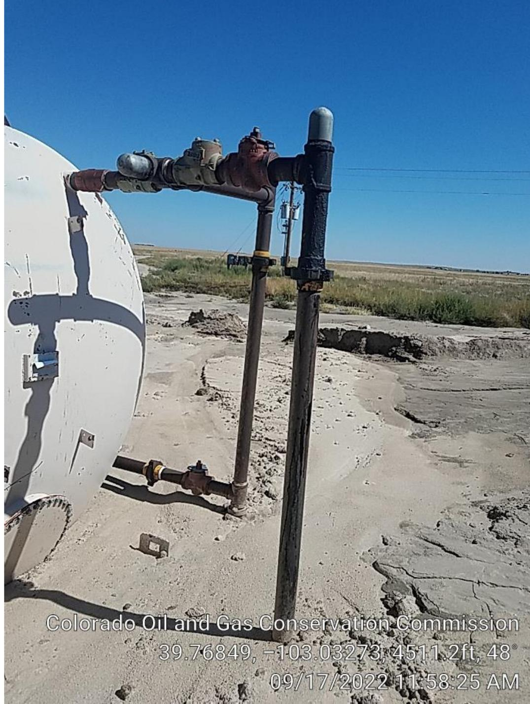
Secondary containment berms around treater/FWKO and produced water tanks to the east are breached.
