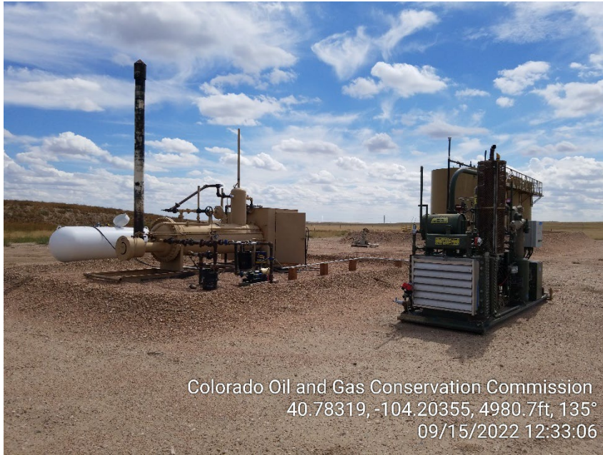
Photo 3 – Separator and Compressor
