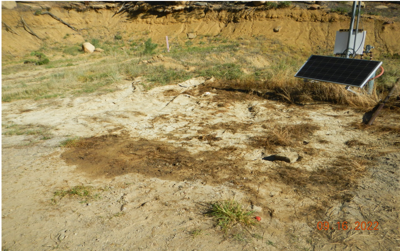
Photo 4. There are additional areas of spills that had occurred. All stained soils need to be cleaned up and properly disposed.
