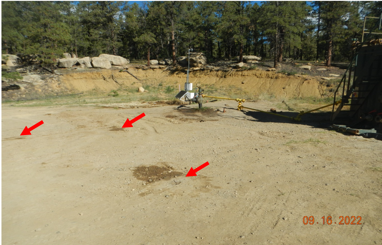
Photo 2. Facing toward the wellsite. There are multiple areas of oil stained soils that need to be cleaned up.
