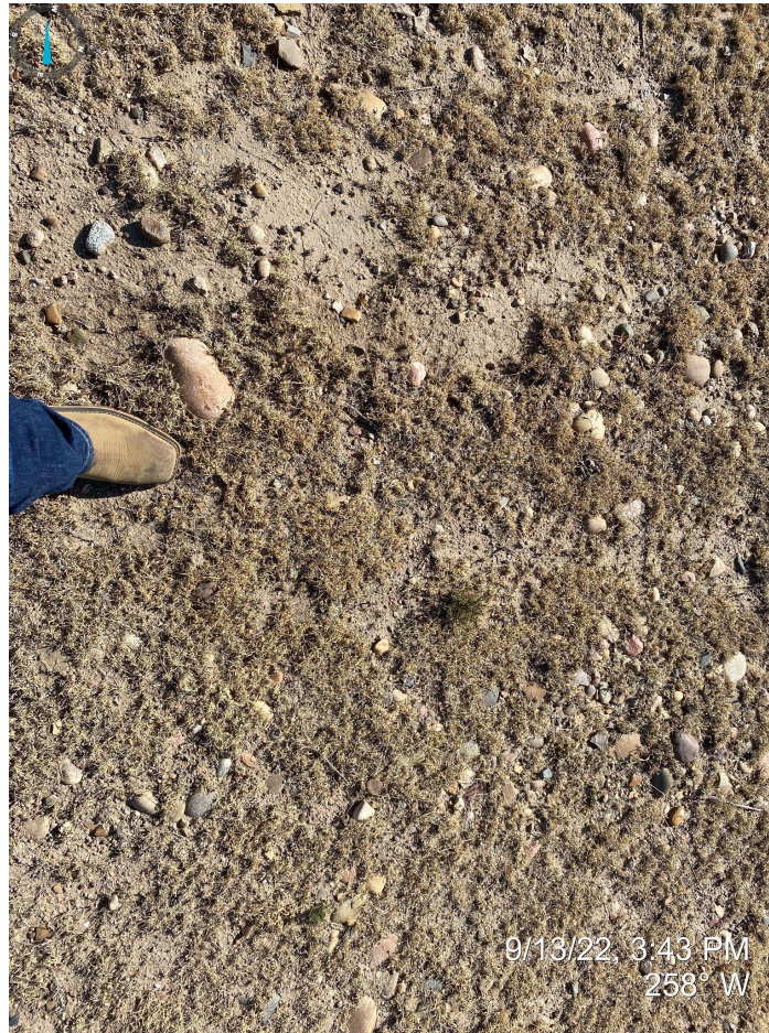
Photo 2. Close up photo of gravel/cobble/road base on access road, illustrating the access road has not been reclaimed.
