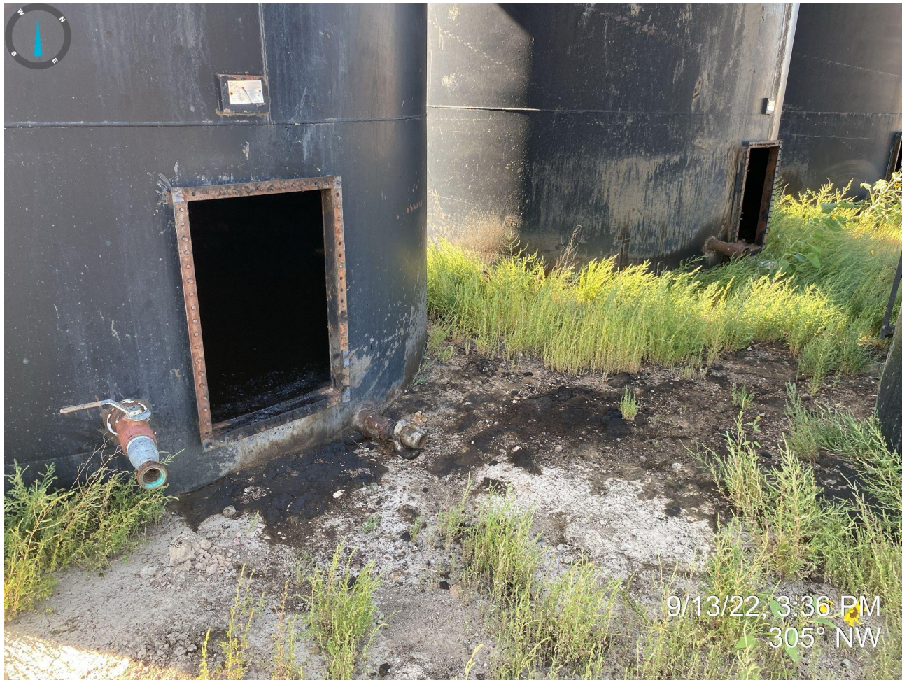
Photo 8. Close up photo of tank batteries with missing manhole covers and oily stained soils.
