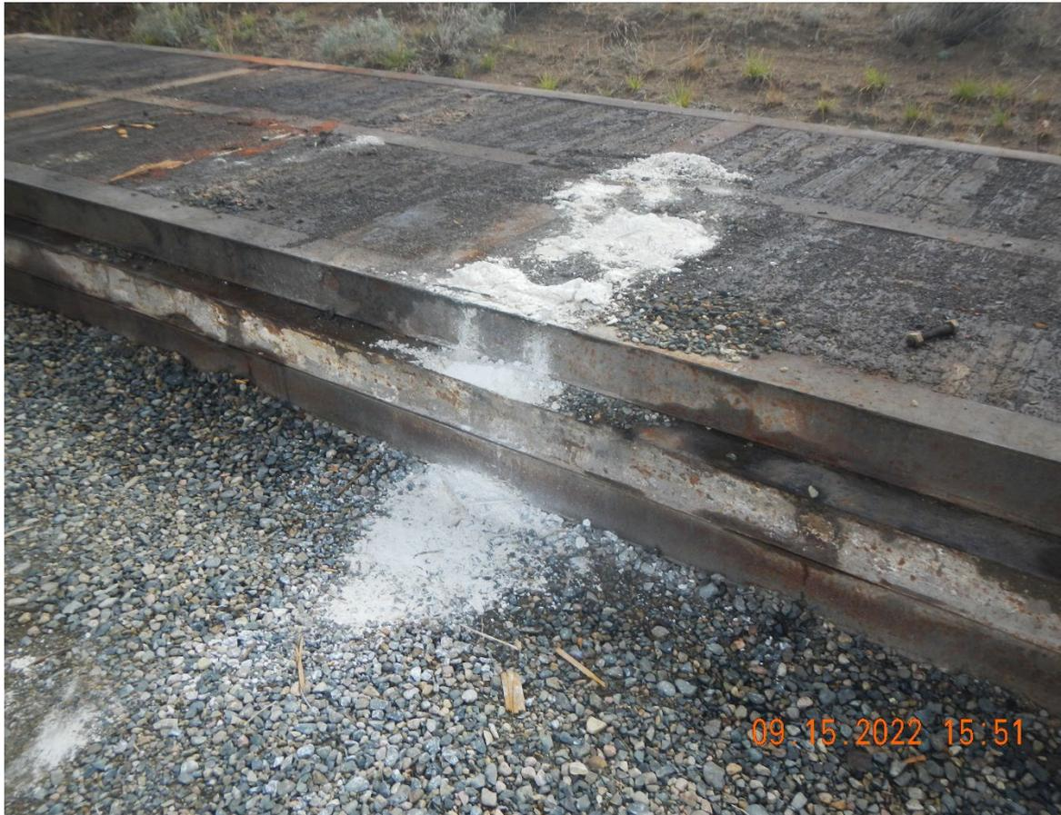
Photo #4 chemical spill on rig skid on south side of pad
