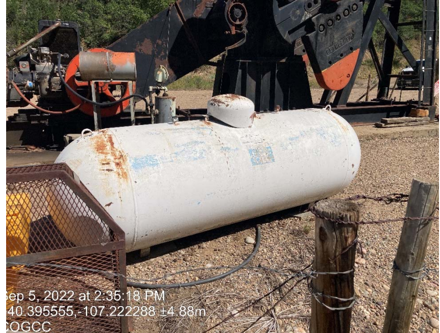
Propane tank lacking labeling
