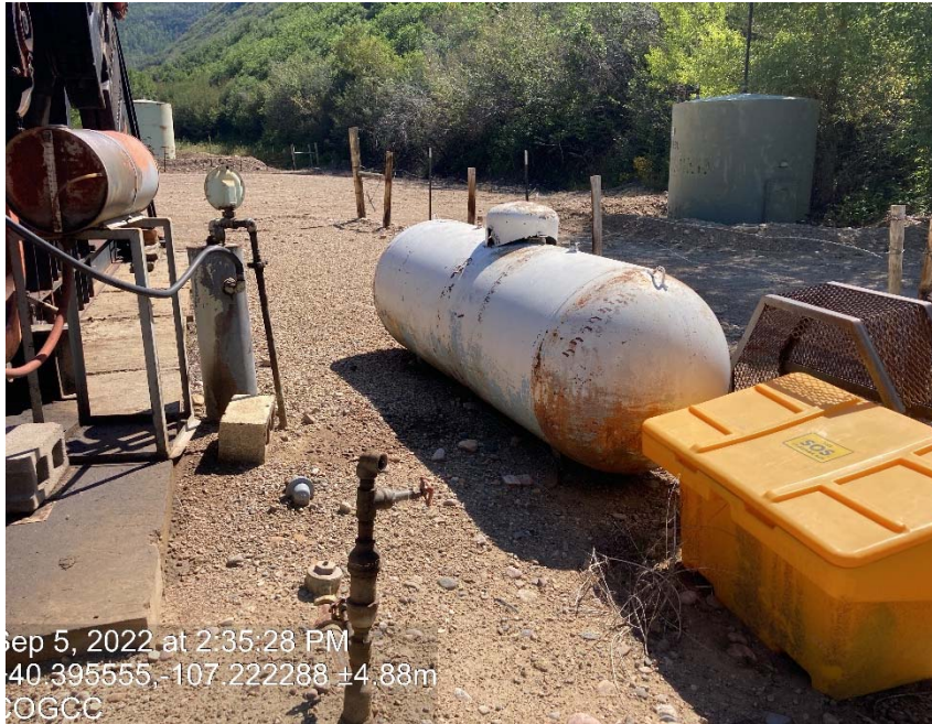
Propane tank lacking labeling
