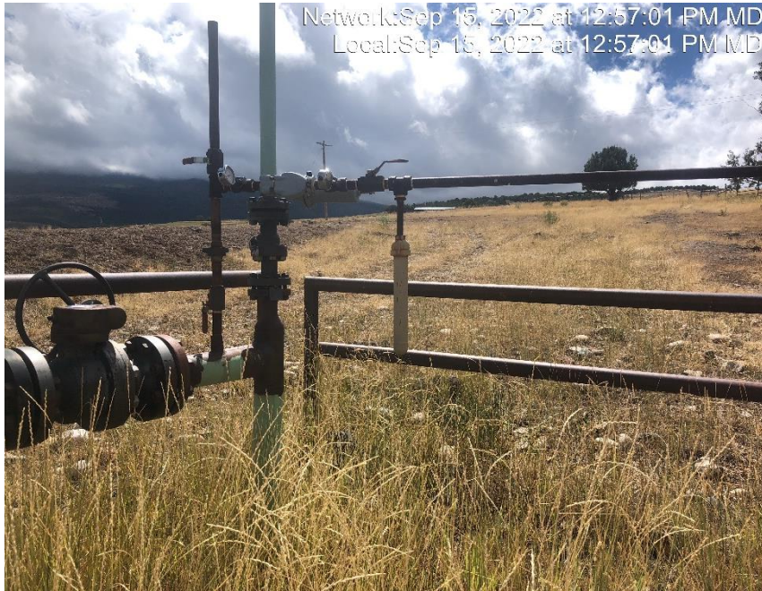
Photo #7703 Domestic tap is derived from TEP sales line.
