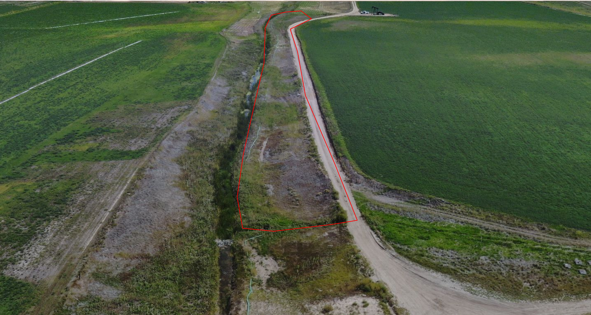
Photo 2. COGCC drone aerial imagery taken on September 13, 2022 documenting the scope of reclamation work to be performed. This image is the approximate extent of reclamation along the western and central project area.
