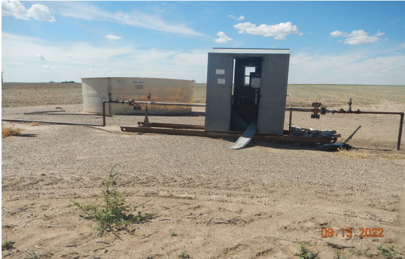
Photo 1. Facing east toward the location. The door to the meter shed is in disrepair and laying on the ground.
