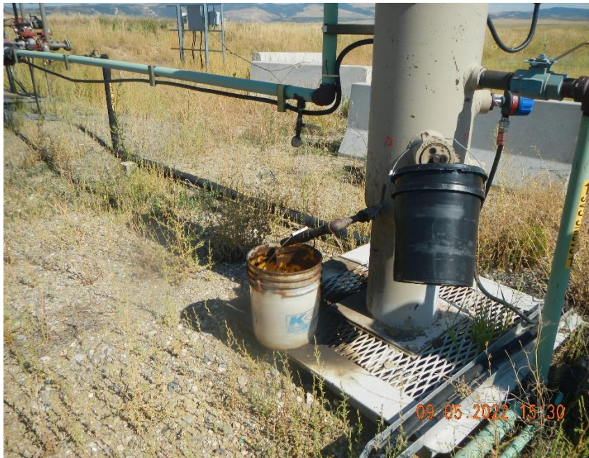
Impacted soils observed around the production equipment at the north of the Location. The containment device at the spill at the north of the Location was observed to be insufficient.
