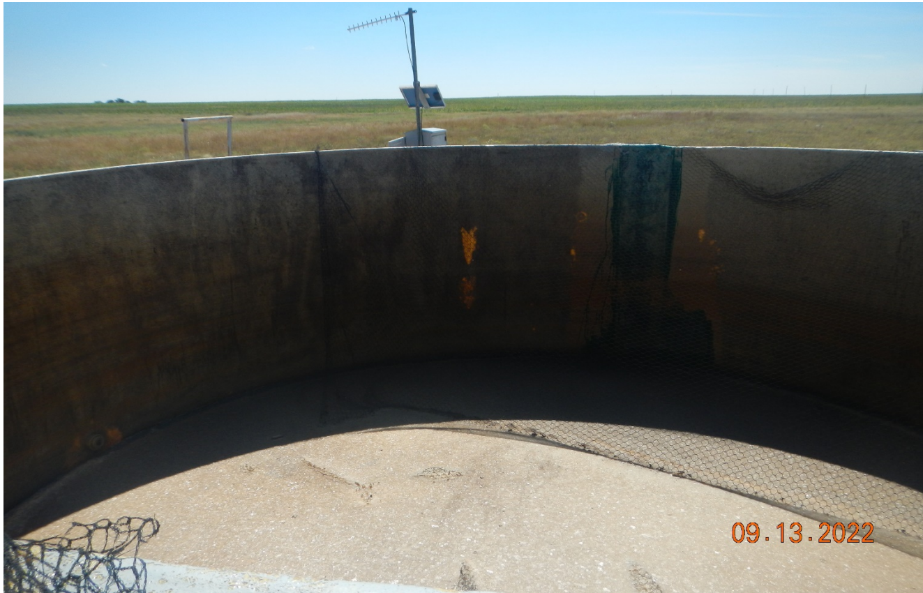
Photo 3. The netting on the tank is in disrepair. Netting needs to be installed to prevent wildlife entry.
