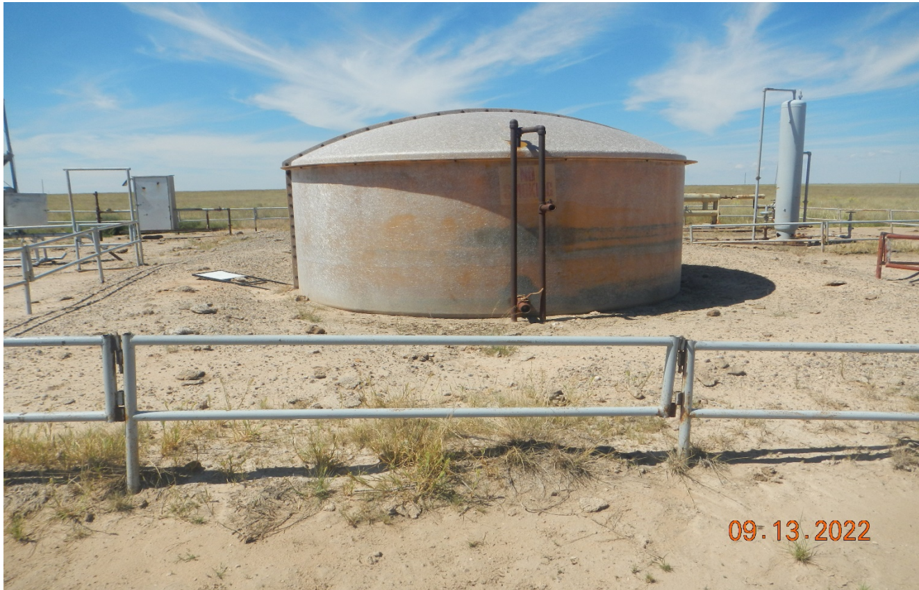
Photo 6. There is no labeling on the fiberglass tank and no secondary containment.
