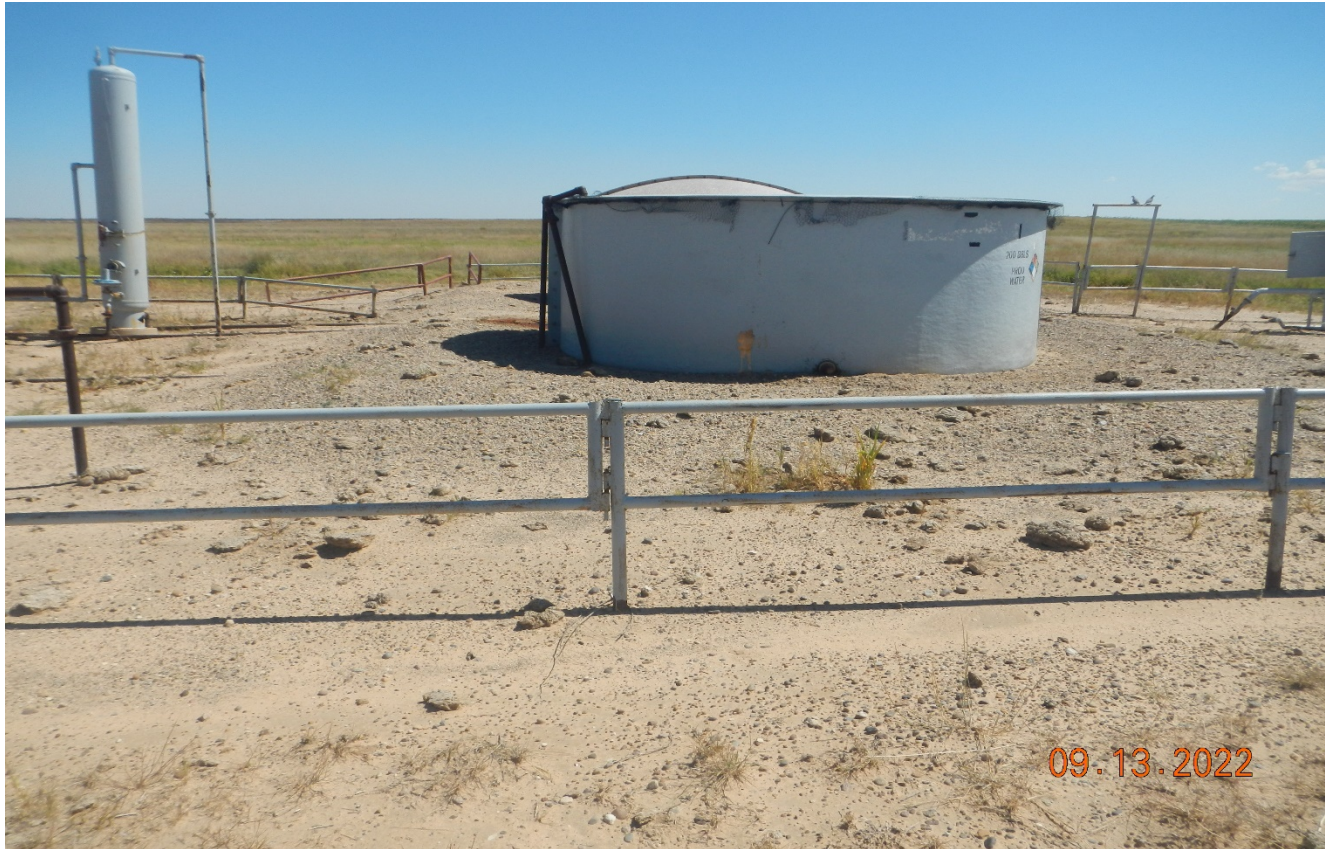
Photo 2. Facing toward the open top tank. There is inadequate secondary containment around the tanks.
