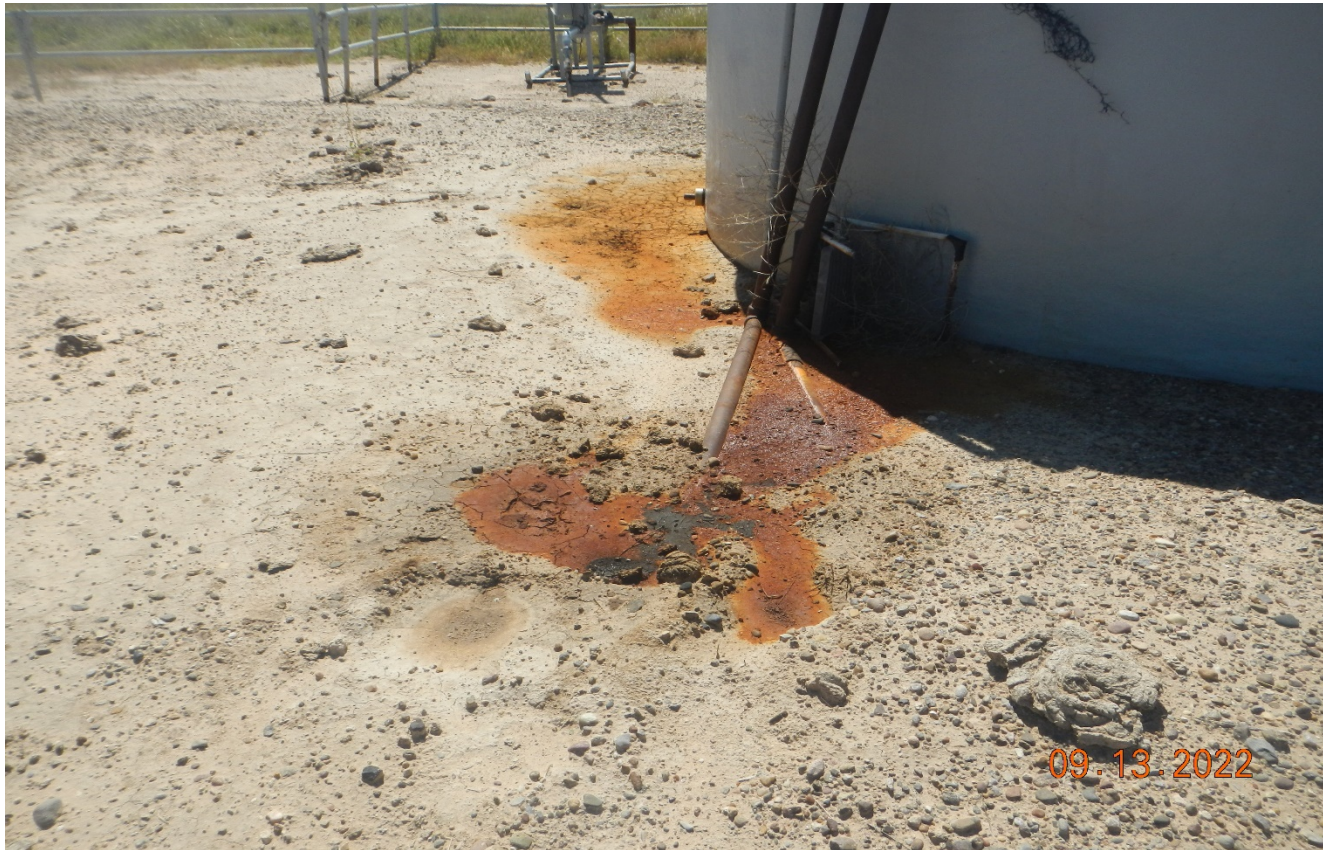
Photo 4. There are signs of a leak that had occurred, perhaps from the piping. Stained soil needs to be cleaned up and the tank and piping need to be inspection for integrity.
