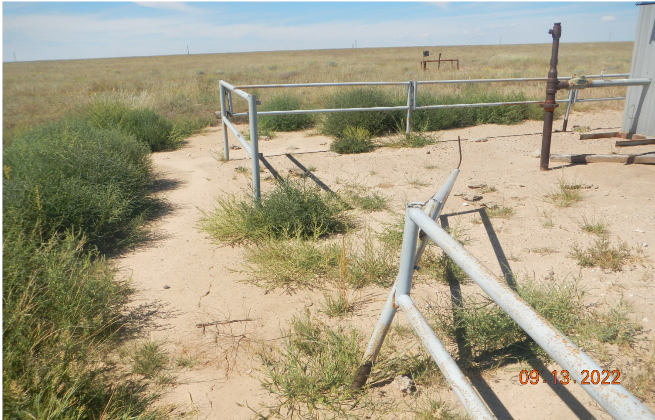
Photo 7. The pipe fence around the equipment is in need of maintenance.
