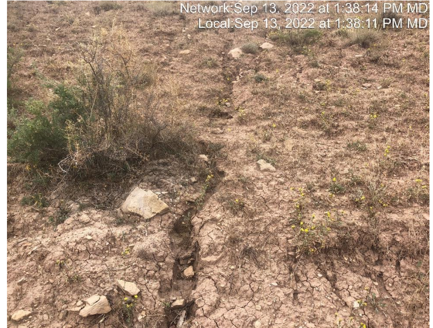
Photo #7680 Rill erosion occurring on cut slope.
