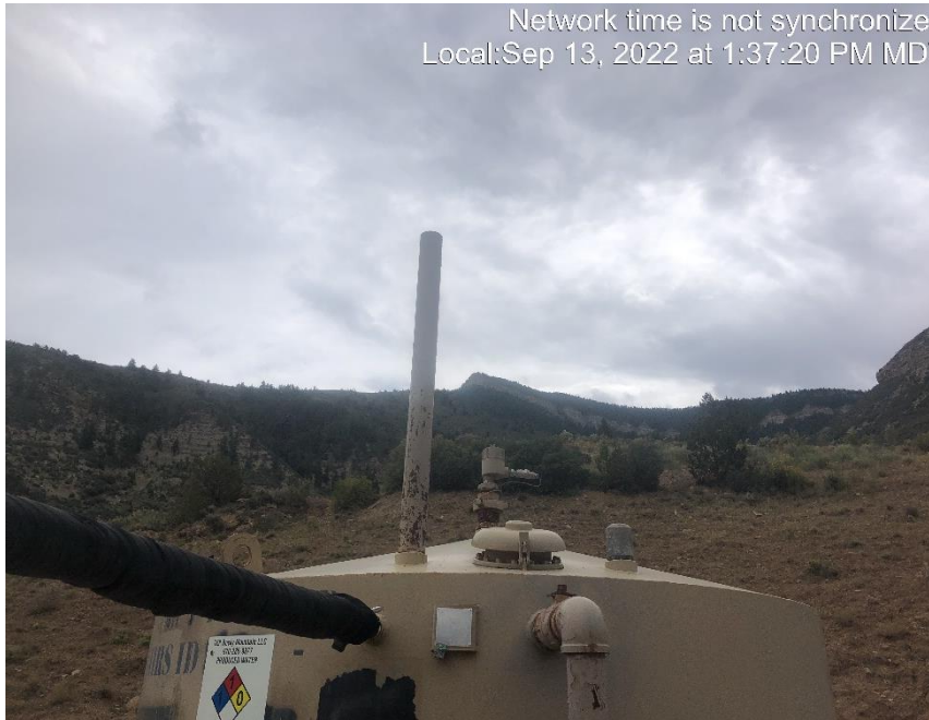
Photo #7677 Vent pipe on tank open ended.
