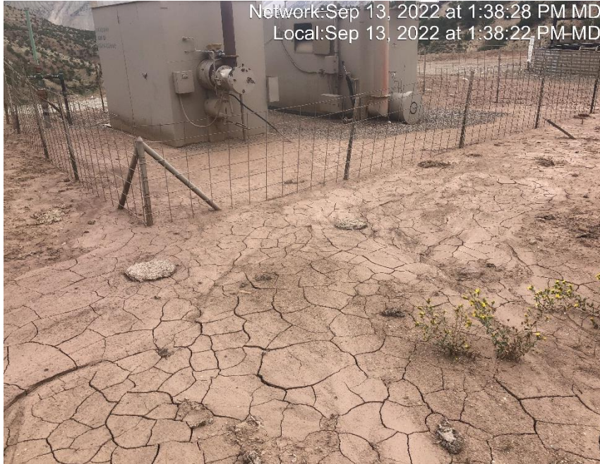
Photo #7681 Sediment encroaching on equipment.
