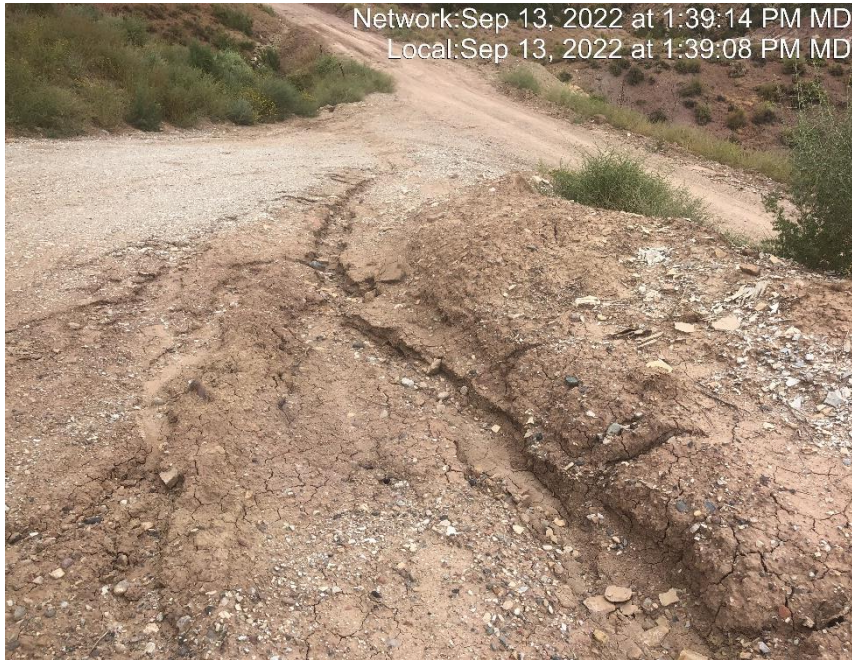
Photo #7683 Rill erosion occurring on access road.
