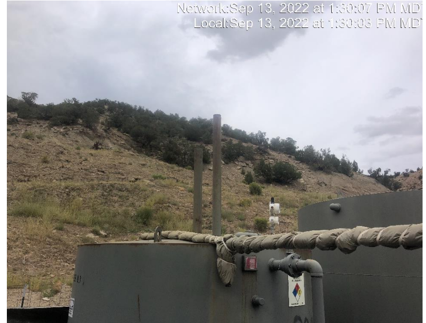
Photo #7671 Multiple vent pipes on tank open ended.
