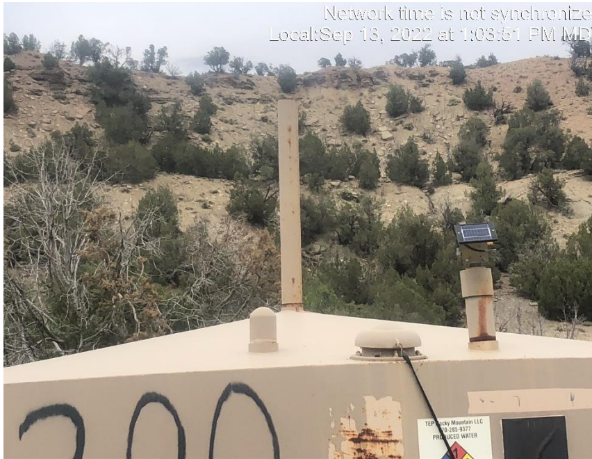
Photo #7654 Vent pipe on tank open ended.
