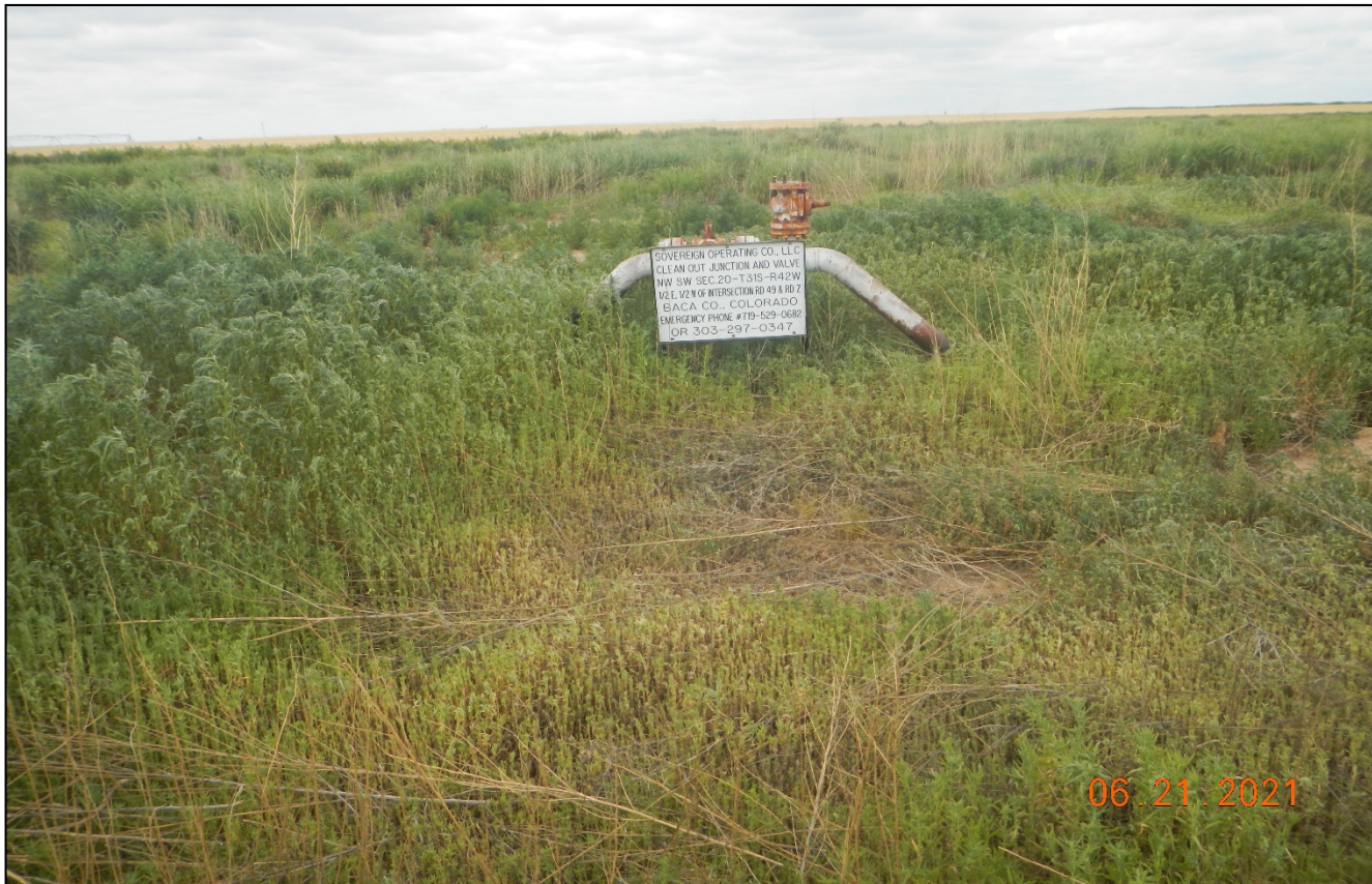
Photo 7. There is a cleanout junction 1850 ft. north of the pipeline which is associated with the former gas compressor station and must be removed.
