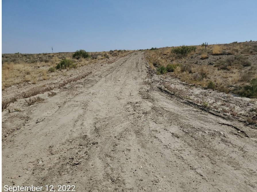
Photo 5: Photos 5-6 taken from access road. Photos show BMPs to minimize erosion, degradation and sediment transport are missing or insufficient along the access road; erosion degradation observed.
