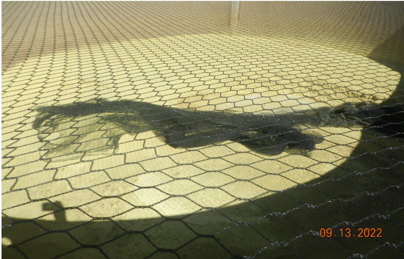
Photo 5. The netting over the tank has been reinstalled.
