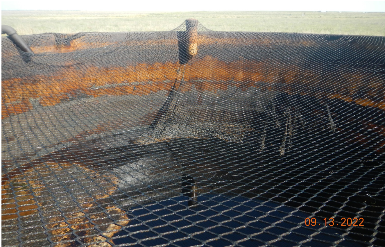
Photo 10. The liquid in the tank has been lowered.
