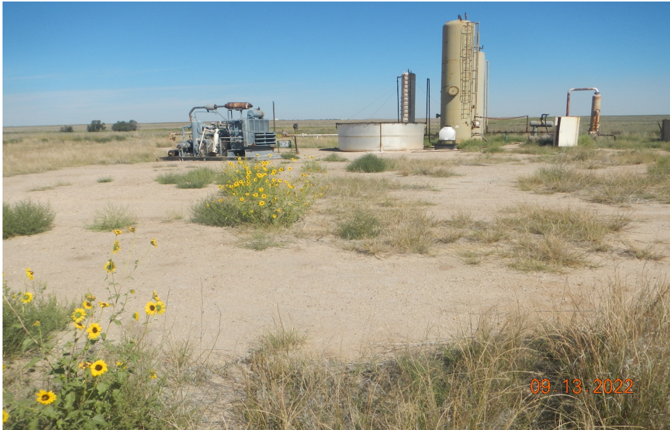
Photo 15. Facing north toward the facility. The surrounding disturbance area has areas that are bare of vegetation that need to be reclaimed per Rule 1003.
