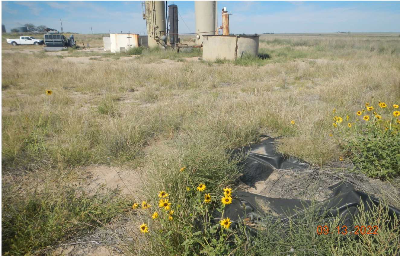
Photo 12. Facing west toward the location. There is a plastic liner debris at east side of the location that needs to be removed.
