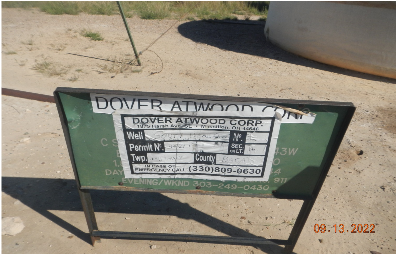
Photo 3. The facility sign is obscured behind the compressor. The sign does not meet the requirements and is not legible. Previous corrective action is not completed.
