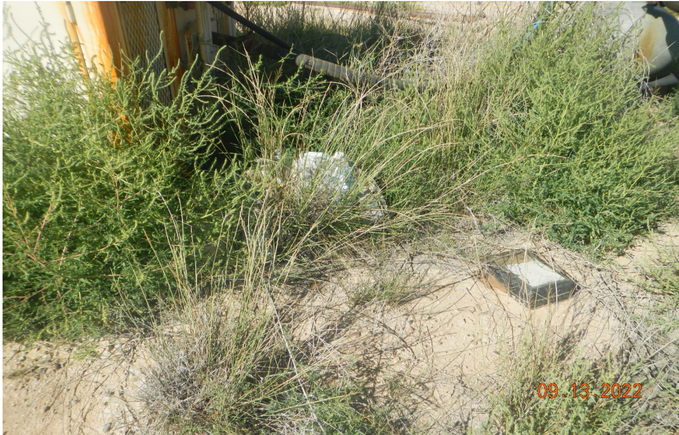
Photo 7. There is oil/chemical containers and trash not properly or disposed of. Previous corrective action is not completed.
