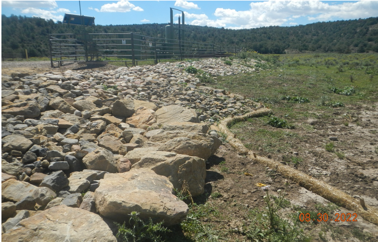
Photo 9. Facing southwest at the west side of the location. Further along the bank the rock rip/rap changes to round rock which does not hold in place very well for proper stabilization. There are numerous noxious weeds in this area that need to be controlled. (Musk thistle, Hounds tongue, Canada thistle).
