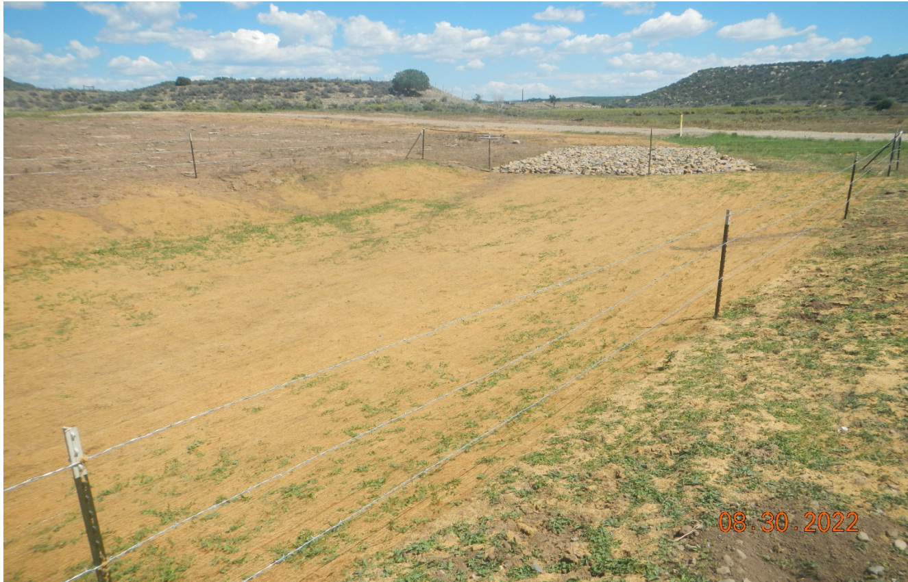
Photo 11. Facing east toward the swaled area at the north side of the location. There has been rock rip/rap, wattles, and erosion blanket installed in this area where erosion had occurred.
