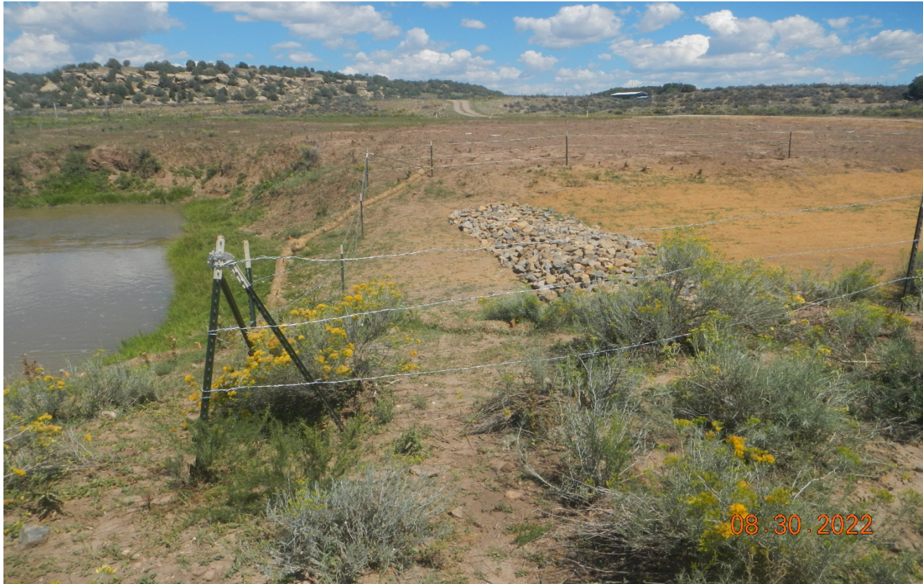
Photo 10. Facing northeast toward the swaled area along the stream bank. There has been rock rip/rap, wattles, and erosion blanket installed in this area where erosion had occurred.
