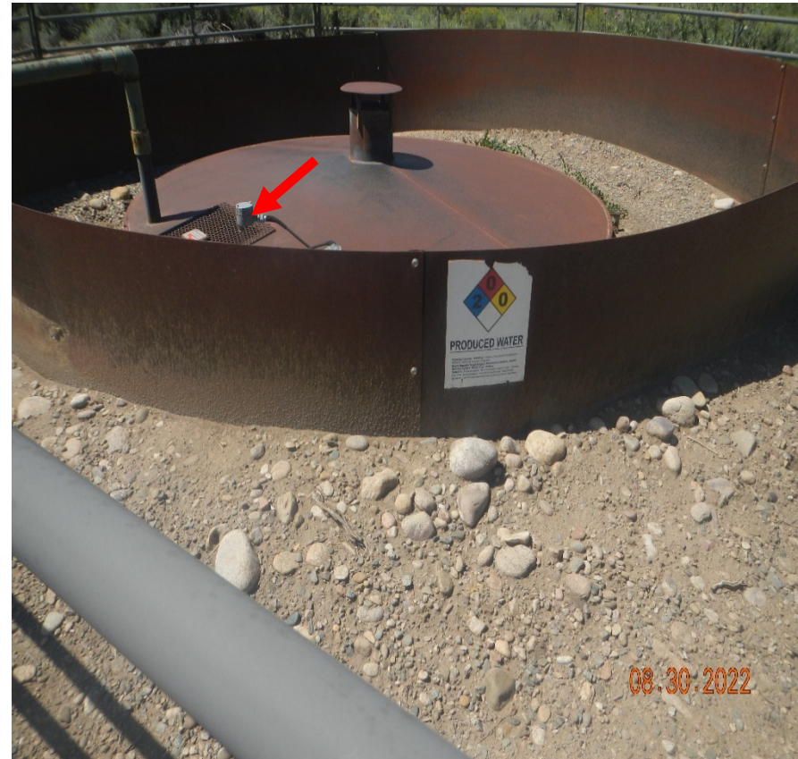
Photo 7. The tank has a steel pervious grate shown at red arrow. This needs to be covered to prevent overflow spillage.
