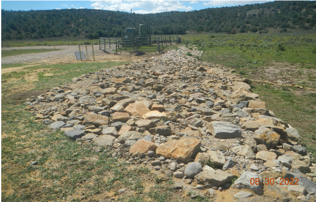
Photo 8. Facing southwest at the west side of the location. This area of previous erosion was repaired and angular rock rip/rap has been installed.
