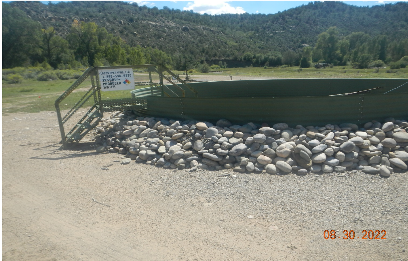
Photo 2. Facing toward the open top tank. There has been round rock placed around the containment. The round rock is pervious and will not prevent flood water from entering underneath the steel containment. Round rock will also be easily displaced as they do not lock in place as well as angular rock. Another solution needs to be implemented.
