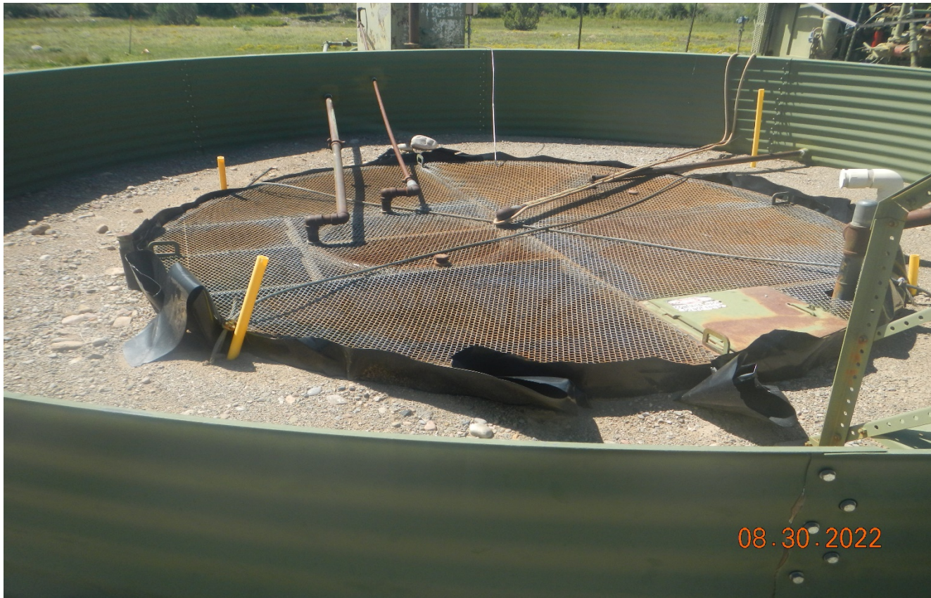
Photo 4. The open top tank has a steel grate which will not prevent spillage from occurring.
