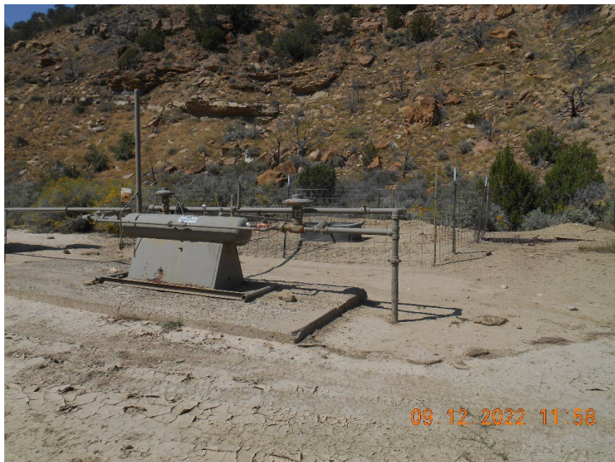
Separator with blowdown tank
