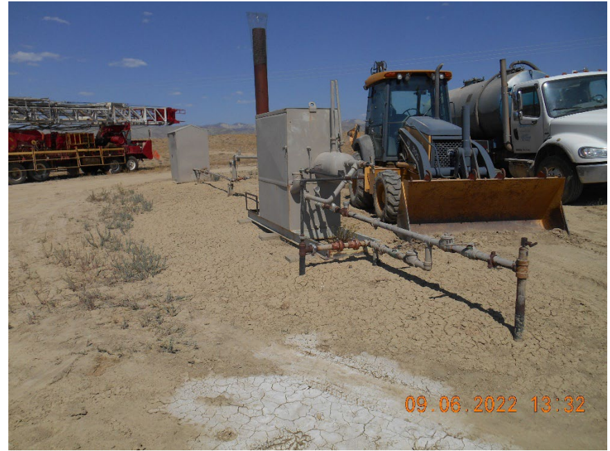
Separator and Meter housing
