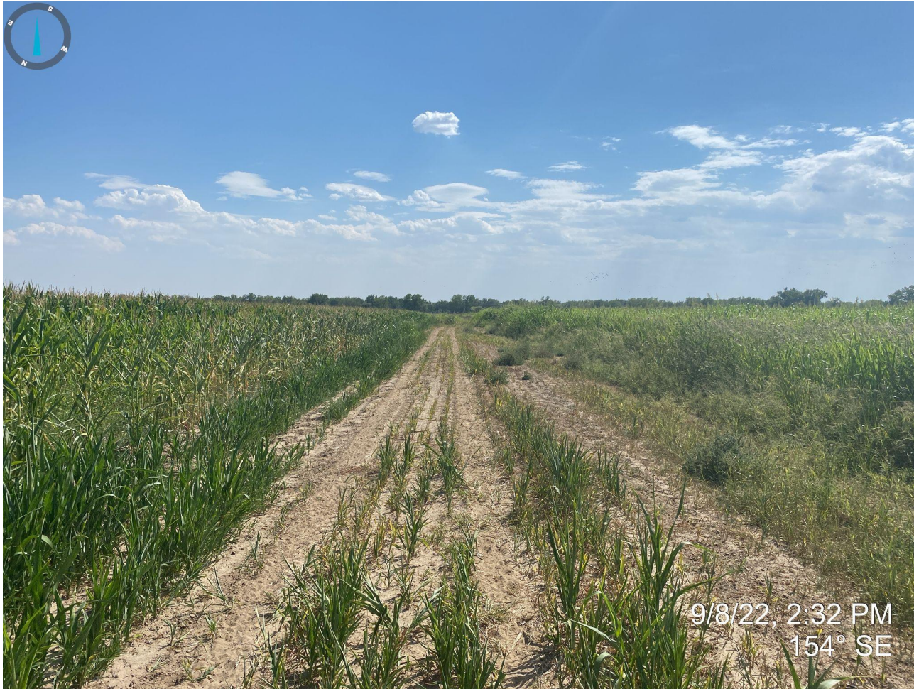
Photo 1. Access road photo taken from county road, facing southeast. Photo illustrates access road has not been reclaimed with presence of bare soil.
