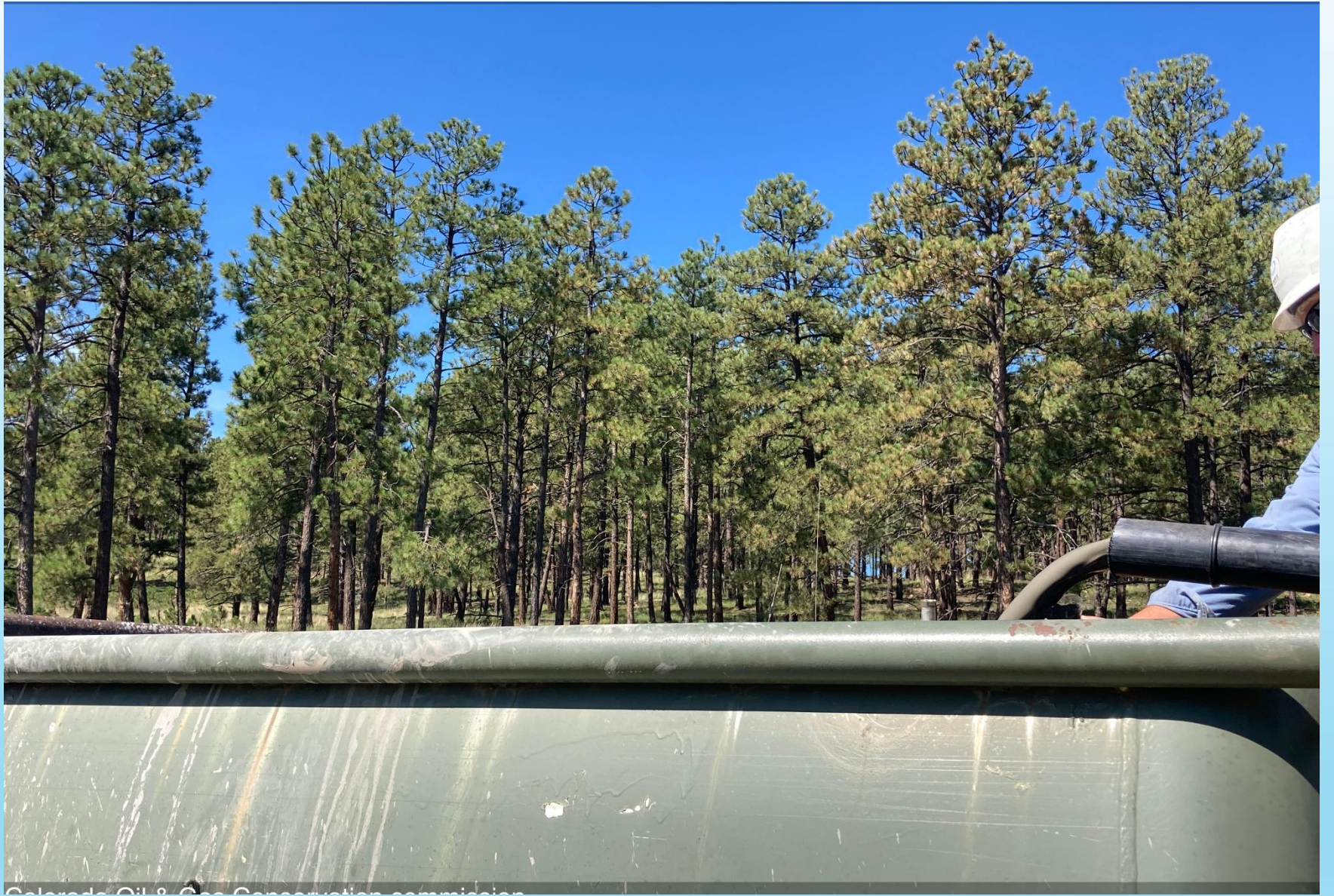
PHOTO 3: GOOD CEMENT RETURNS TO SURFACE TANK.
