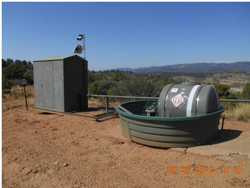
Meter housing. Secondary containment of chemicals
