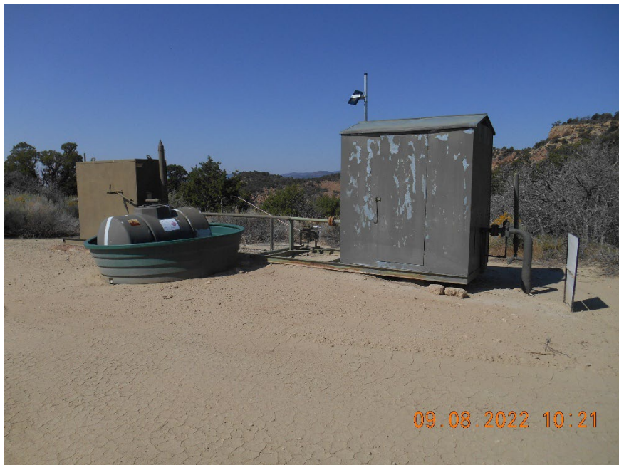
Separator and Meter housing. Secondary containment of chemicals
