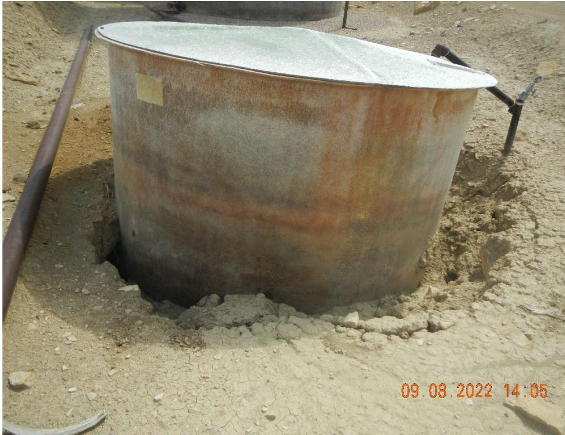
**Photo #3 partially buried tank is heaving and would allow fluid to the subsurface in case of a spill.**
