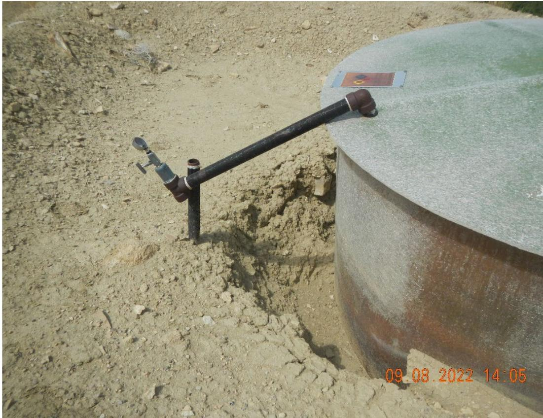
**Photo #4 partially buried tank is heaving and would allow fluid to the subsurface in case of a spill. It appears that the tank is not piped, if tank is not necessary, it should be removed.**
