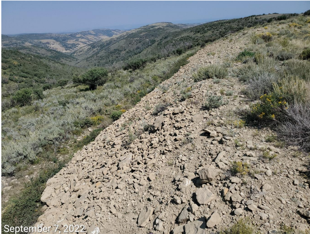
Photo 2: Photo shows bare fill slope; location has not been recontoured/regraded and reclaimed.
