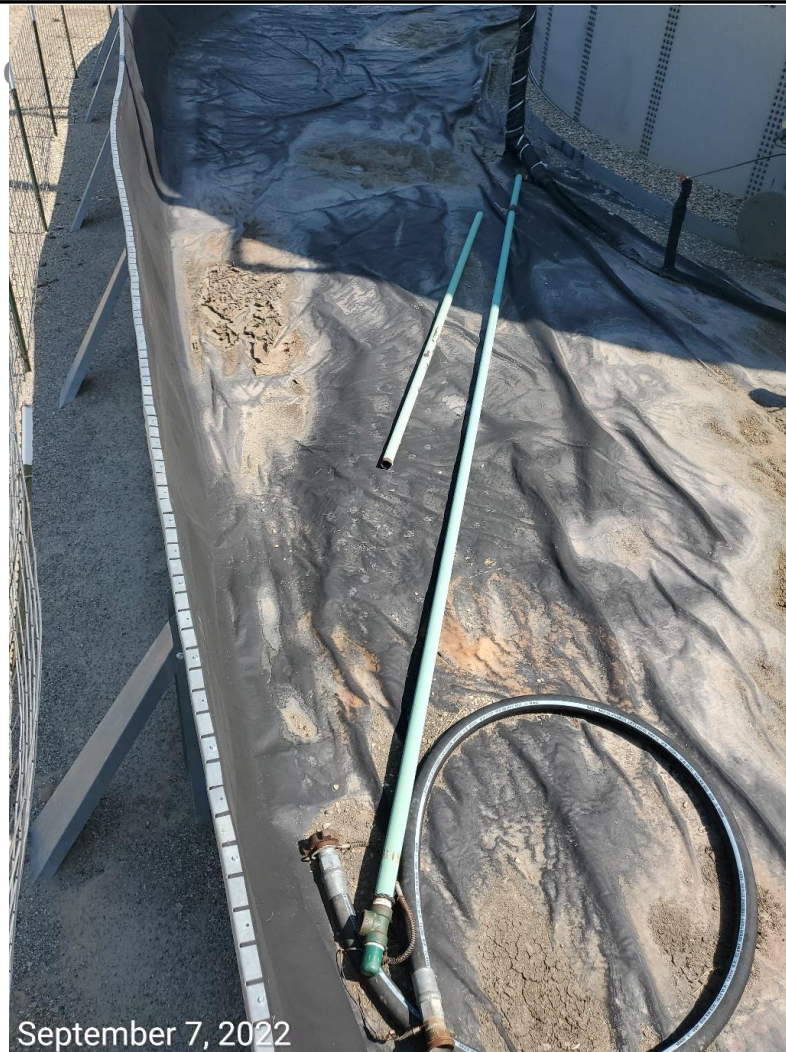
Photo 6: Photo shows unused pipe equipment stored within the secondary containment berm of the tank battery.
