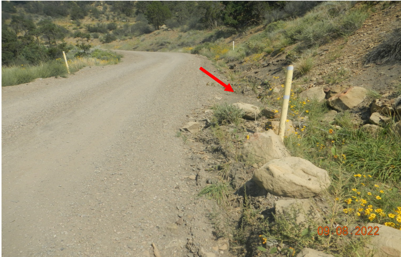
Photo 2. Just past the compressor facility, stormwater is not properly diverted off the road in this area and is flowing past the diversion shown at red arrow.
