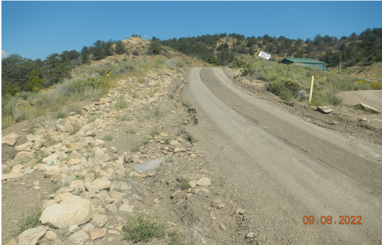
Photo 3. There is erosion occurring at the access road. Which is not being diverted toward the rock rip/rap outlet.
