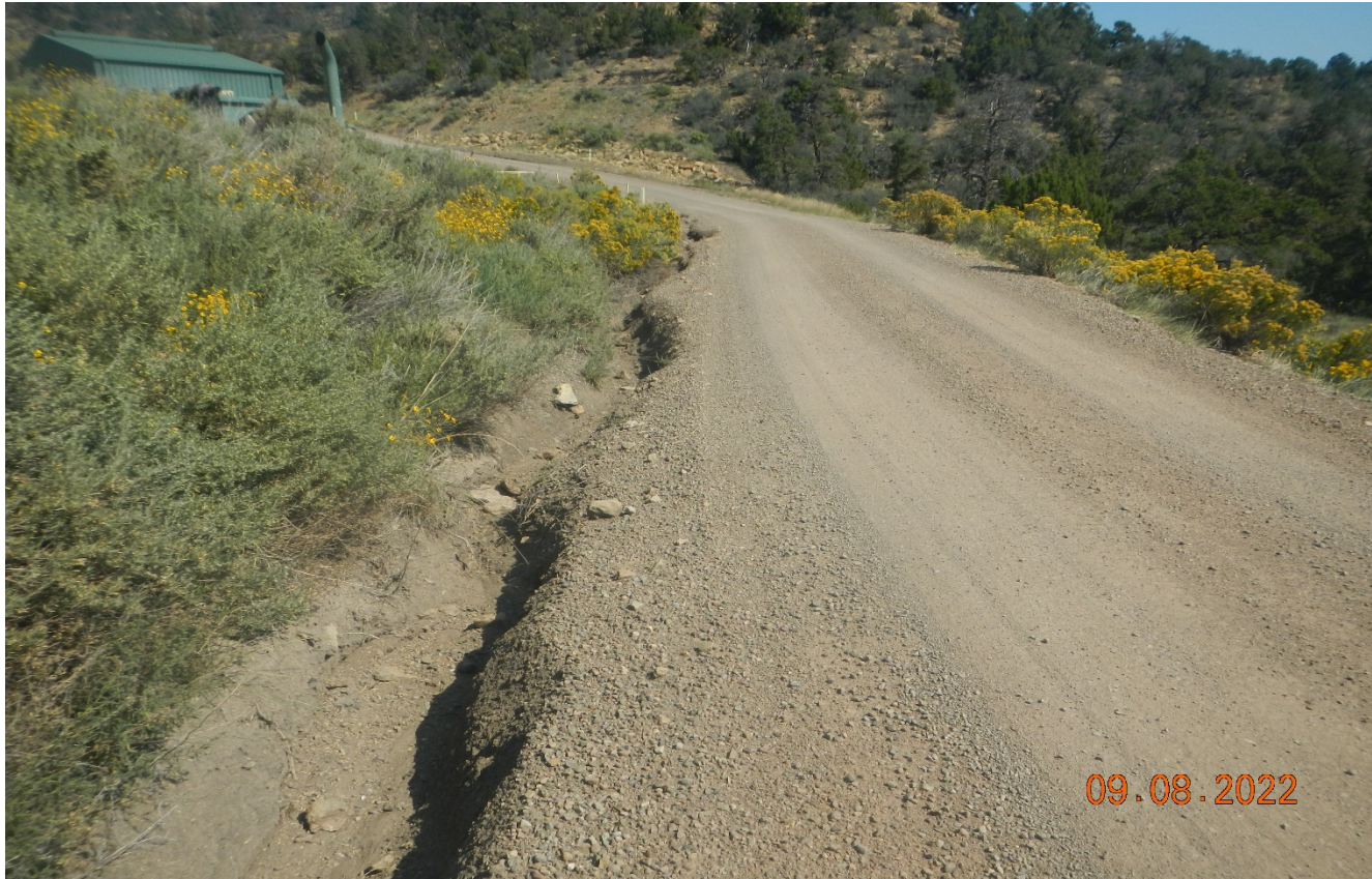
Photo 1. Facing north along the road. The road side is eroding in this area due to concentrated stormwater flow. BMP's need to be installed in this area (e.g. check dams, rip/rap).
