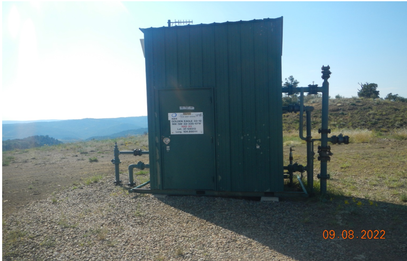
Photo 3. Sign installed at meter shed.
