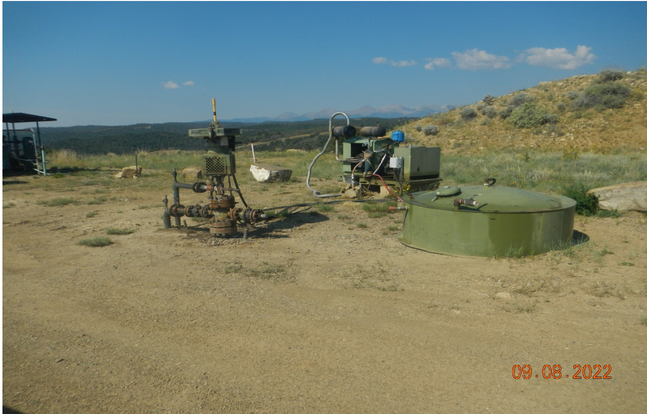
Photo 3. Leak has been repaired.
