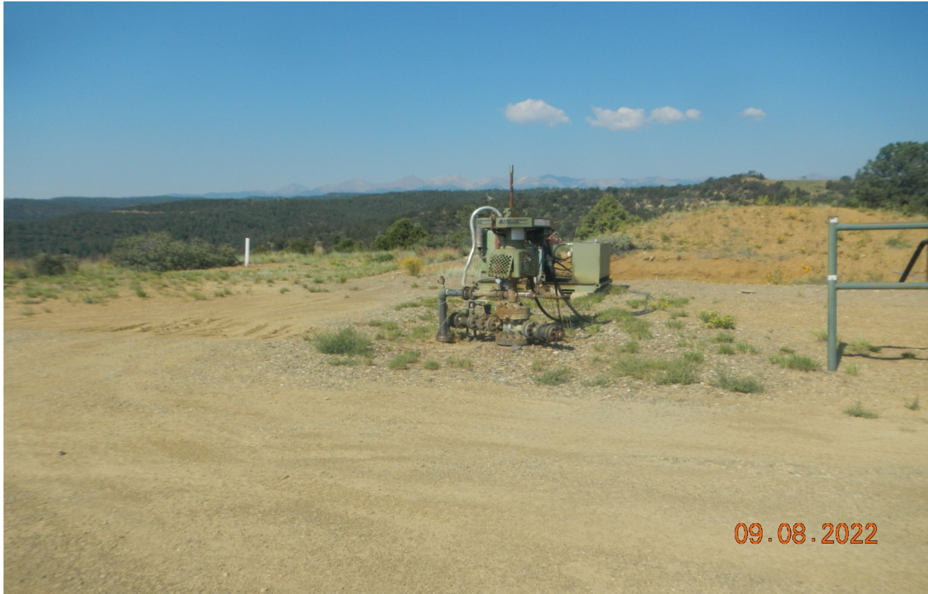
Photo 1. Leak has been repaired.
